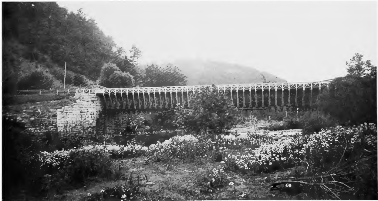
FIGURE 107.—Neversink Aqueduct at Cuddebackville, New York, which had the longest single span of the Delaware & Hudson Canal suspension aqueducts. (Courtesy of Division of Mechanical and Civil Engineering, National Museum of History and Technology, Smithsonian Institution.)
