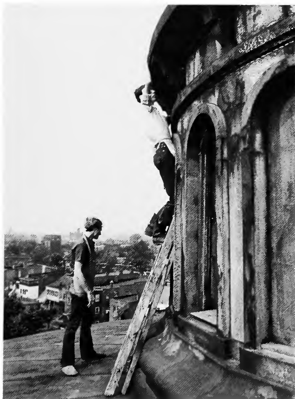
FIGURE 4.—DeLony and Parrott atop the Gasholder House, June 1969. (Vogel)
