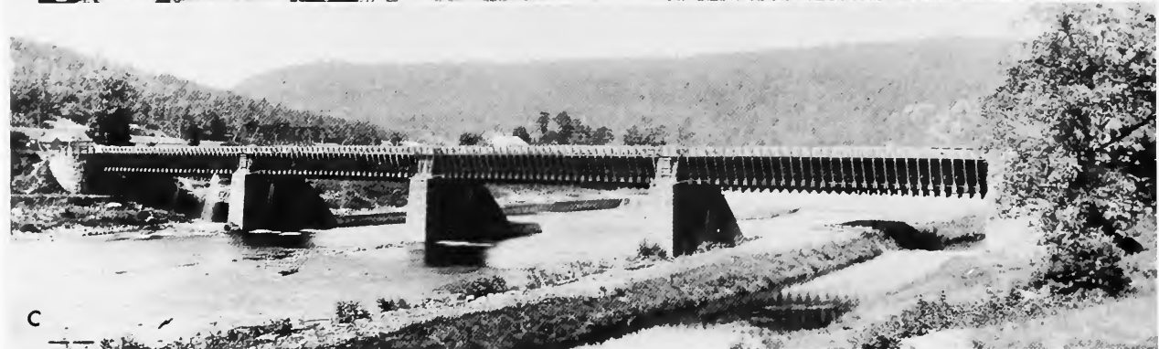
FIGURE 105.— a , Delaware Aqueduct from above the mouth of the Lackawaxen, shortly before suspension of canal operations. The Delaware & Hudson Canal dam, retained after construction of the aqueduct to provide water for the section of the canal to the east, is just in front of the aqueduct piers. b-c , Downstream side of the Delaware Aqueduct before abandonment. Except for the canal's absence, Lackawaxen, Pennsylvania, seen across the river, has changed little over the years. In c may be seen the Erie Railway's truss bridge over the Lackawaxen, the remains of the 1828 canal, and the canal company's dam across the Delaware. ( a : Courtesy of Delaware & Hudson Railway Company; b : courtesy of Jim Shaughnessy; c : courtesy of Delaware & Hudson Canal Historical Society, Gear Collection.)
