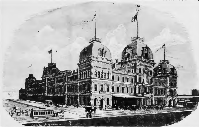
GRAND CENTRAL DEPOT, NEW YORK. IRON WORK CONSTRUCTED BY ARCHITECTURAL IRON WORKS.
