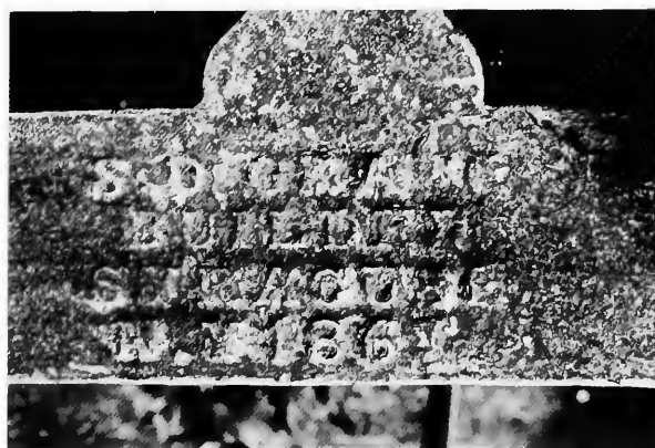
FIGURE 91.—Whipple Truss Bridge, top-chord end casting with builder's inscription.
