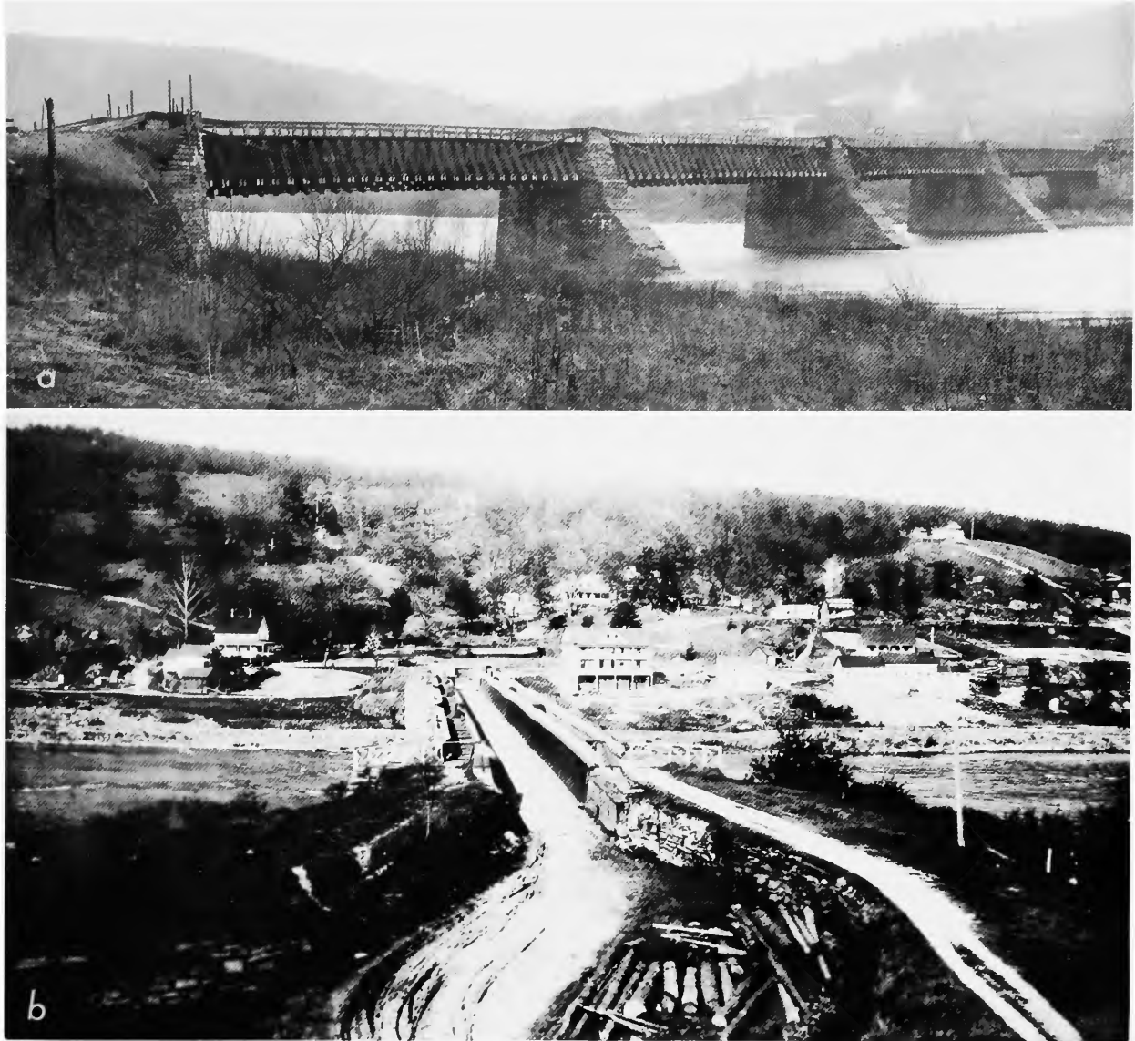
FIGURE 109.— a , Early twentieth-century view of the Delaware Aqueduct from New York; b , the Delaware Aqueduct and Minisink Ford, New York, shortly after the canal's abandonment in late 1898. Except for removing the berm wall on the outside of the curve at Lackawaxen to provide road access, nothing has yet been done to alter the structure for toll-bridge service. (Courtesy of Delaware & Hudson Railway Company.)
