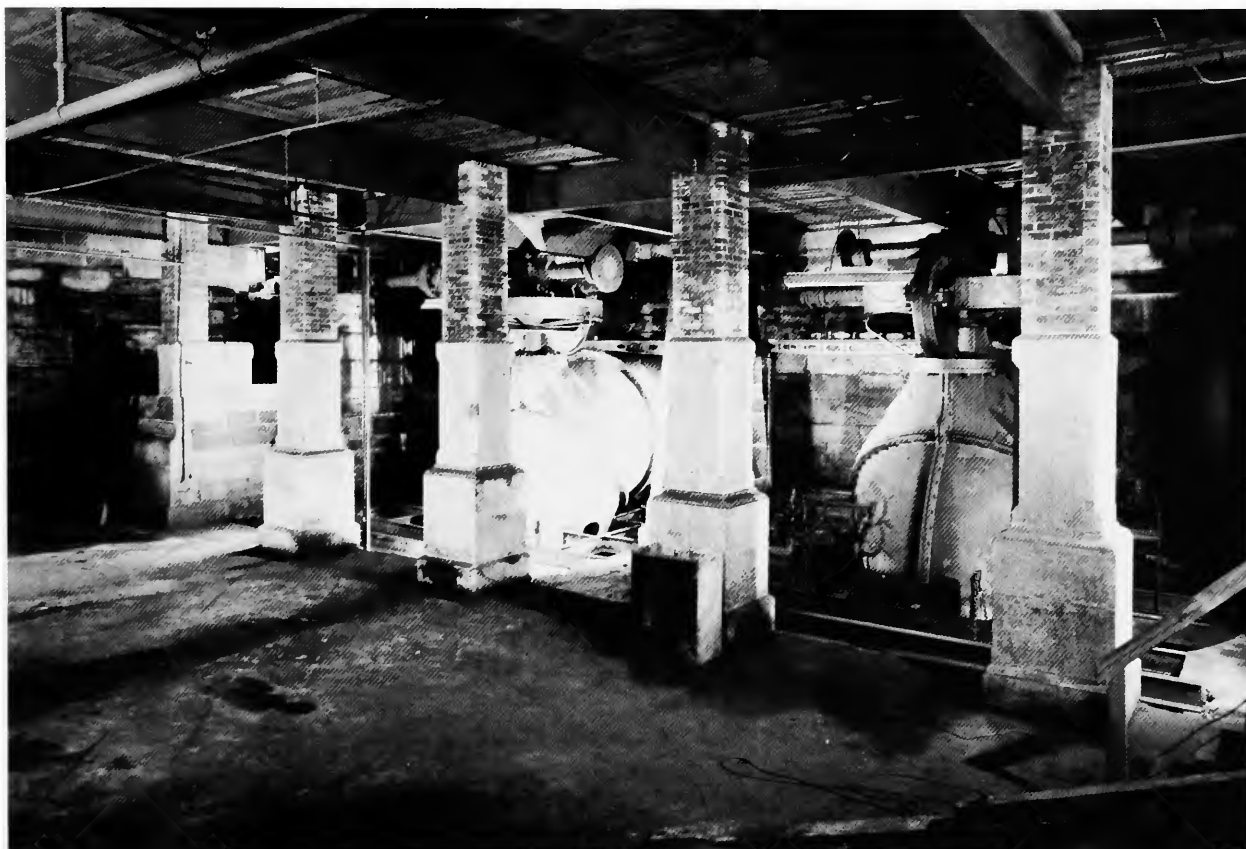
FIGURE 71.—General view of the Holyoke turbines and wheel room, south block in Harmony No. 3 Mill. The installation is original, although the turbine runners (the rotating elements) were undoubtedly replaced several times during their operating life. These units are similar to those installed in the north block, now removed, but were twice as powerful, hence two rather than three units (see Figure 66a). The cast-iron service bridges between the turbines were for oiling the main bearings and the gears.
