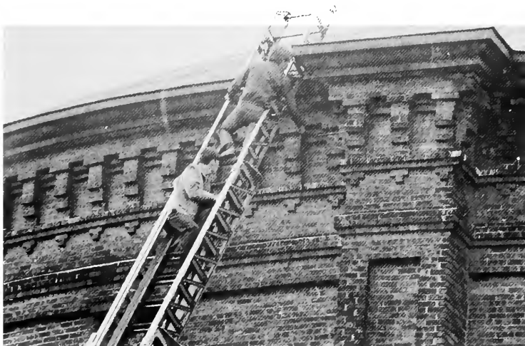
FIGURE 3.—M-HAS team members Parrott and Bouse measuring cornice of the Gasholder House from an aerial ladder truck furnished by the Troy Fire Department, June 1969. (Pollak)
