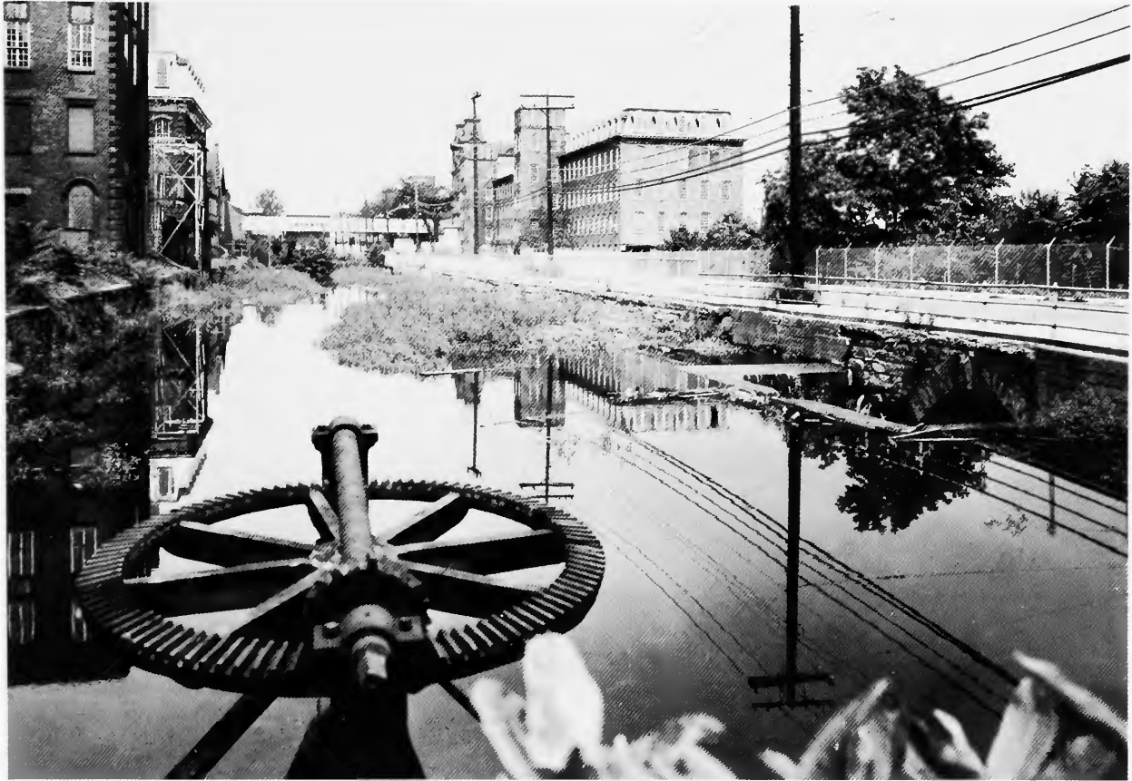
FIGURE 77.—View north along the second level canal, Harmony No. 2 Mill on left; No. 3 Mill on right.
