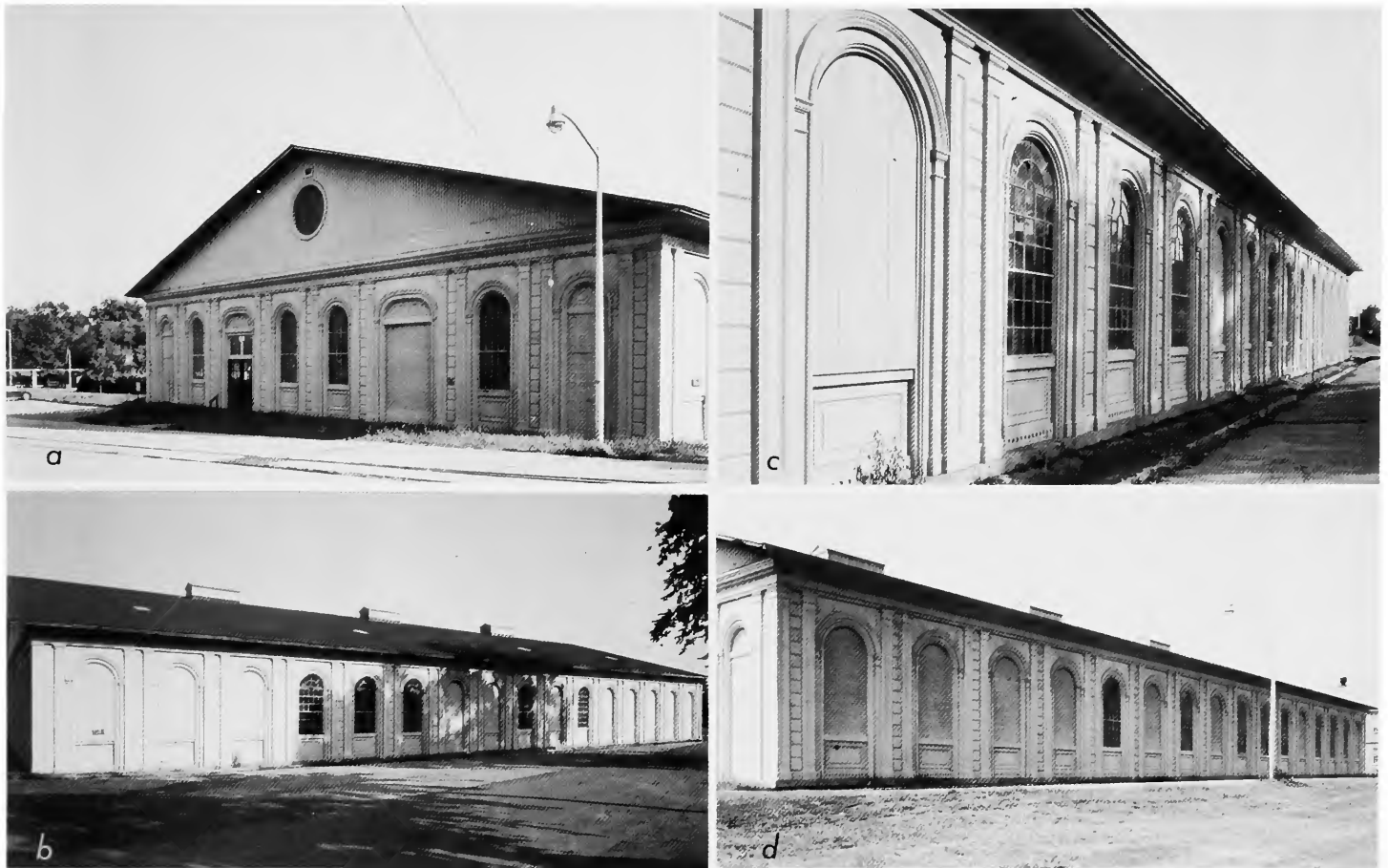
FIGURE 21.—Storehouse: a , North elevation; b , west elevation; c , detail of west elevation from the northwest; d , east elevation from the northeast.
