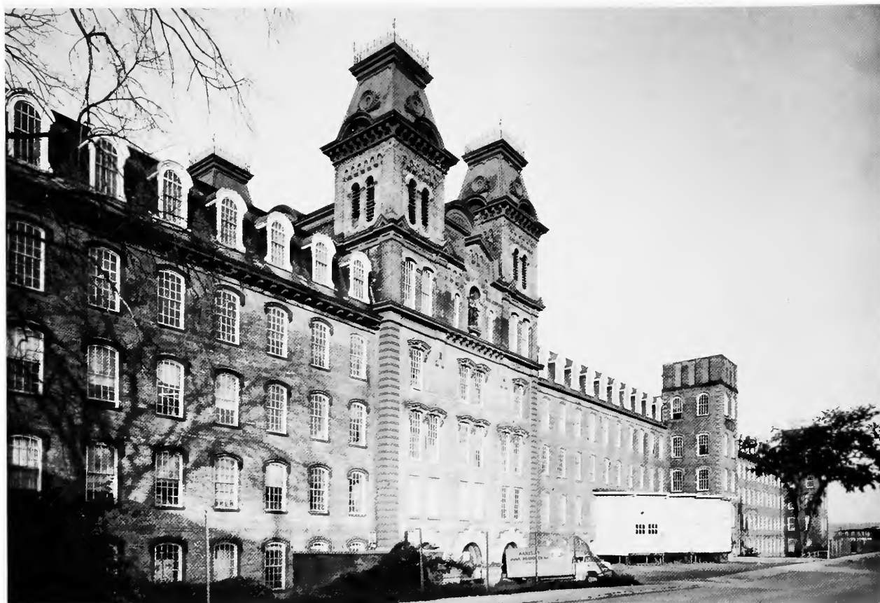
FIGURE 68.—Principal face of the Harmony No. 3 Mill from the northwest: central and south blocks.
