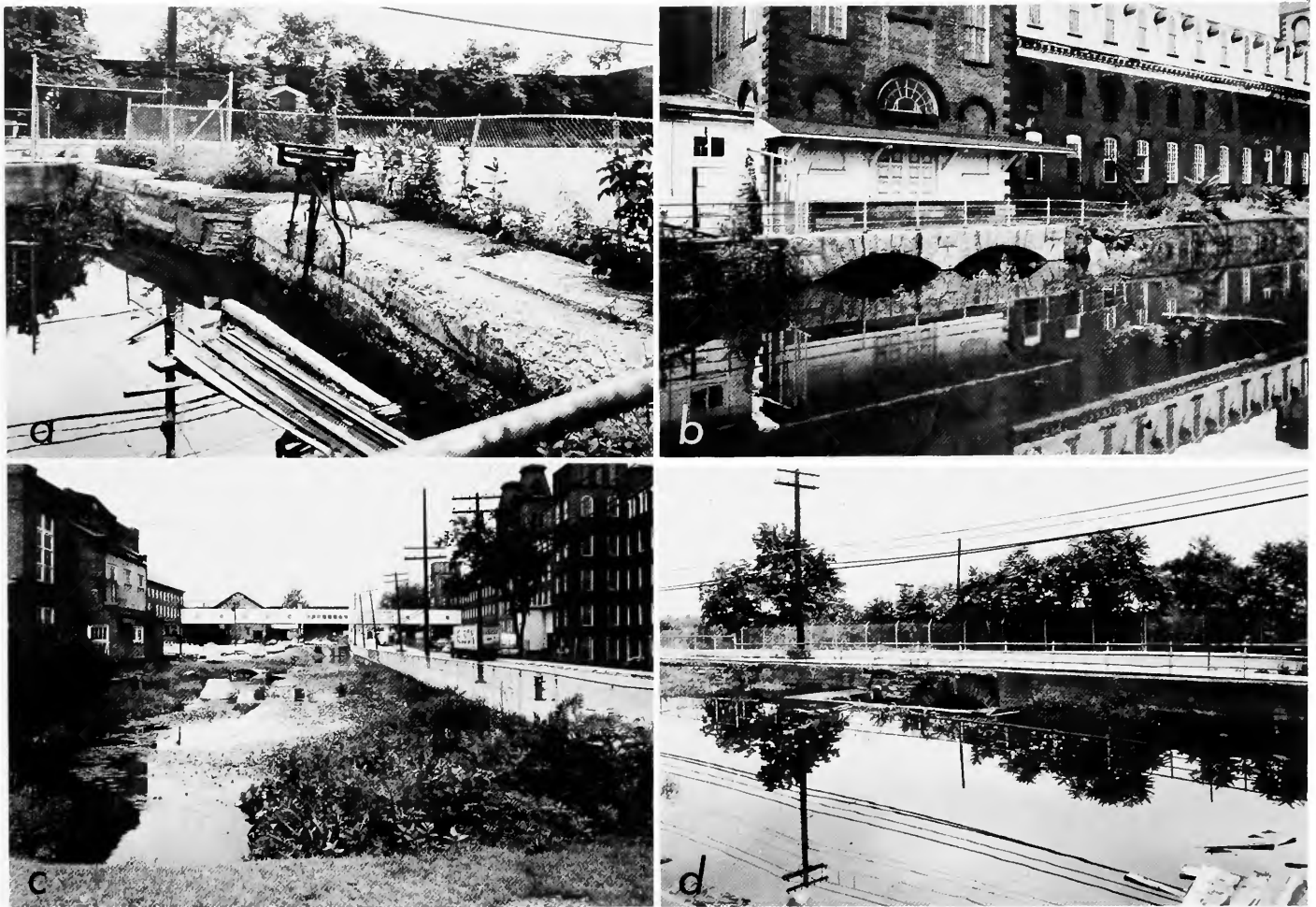
FIGURE 75.—Second level canal: a , South end, gate control to let water directly into the third level canal; b , arches over intakes at Harmony No. 2 Mill; c , looking north between Harmony Nos. 2 and 3 Mills; d , south end, spillway into the Mohawk River to prevent overtopping of the berm.
