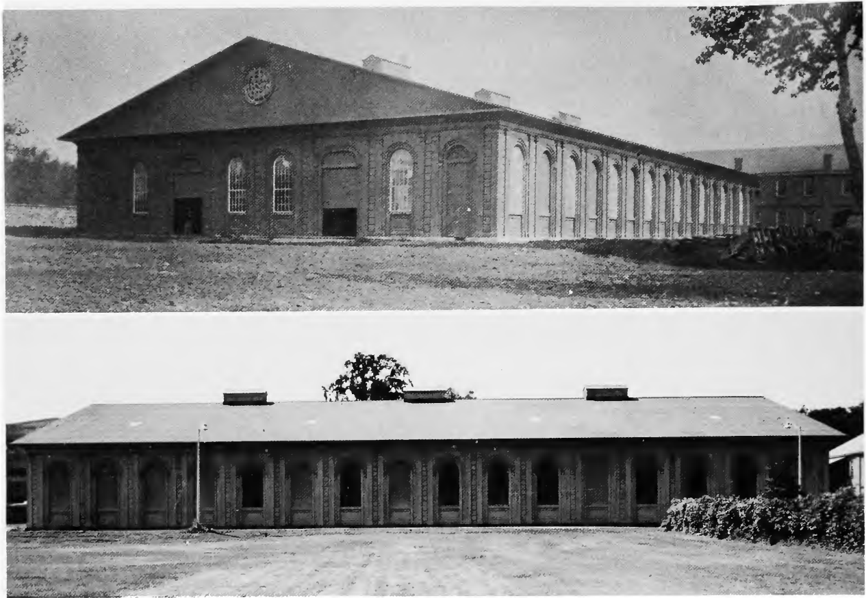
FIGURE 20.—The appearance of the Storehouse has remained practically unchanged during its lifetime: south and east faces, May 1875 (top); east face, August 1972 (bottom). (Top: Courtesy of the Public Information Office, Watervliet Arsenal; bottom: Boucher.)
