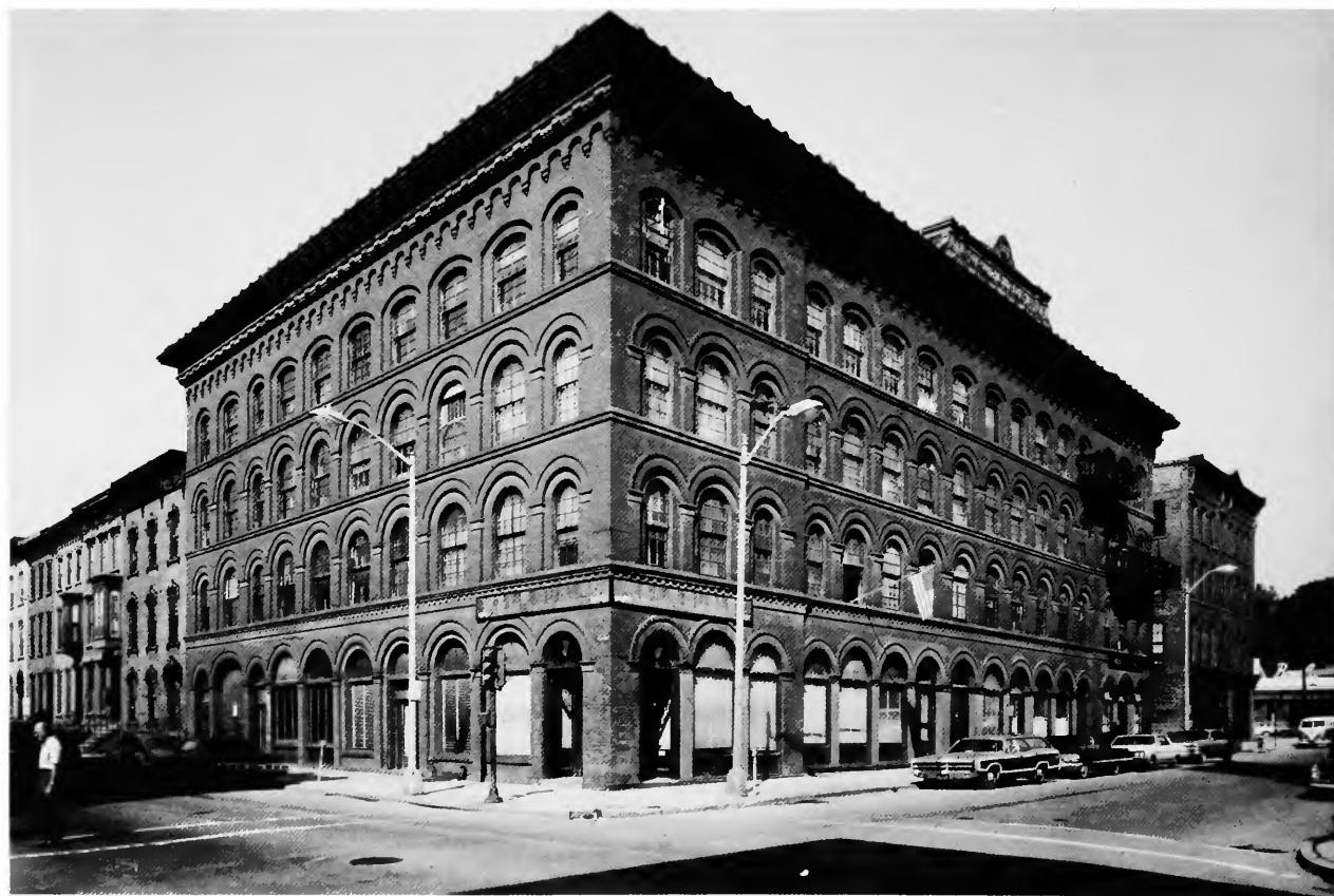
FIGURE 79.—General view of the Gurley Building from the southwest.
