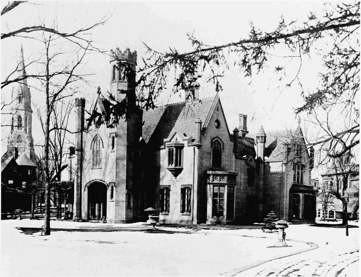
Figure 8. Compared with Davis's plan for an addition to the Harral residence, the library built in 1866—seen in this photograph as the projecting bay at the back of the house—was undistinguished. Fortunately, however, it was compatible with the established architectural style. (Smithsonian negative 68115.)
