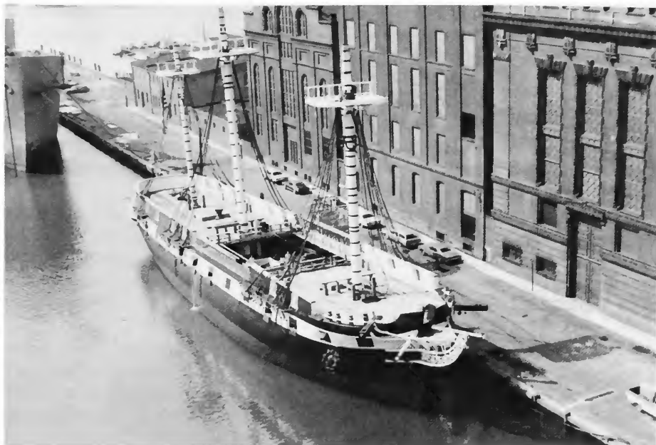
FIGURE 7.— Constellation during present reconstruction at Pier 4, Baltimore, Maryland, August 1968.
