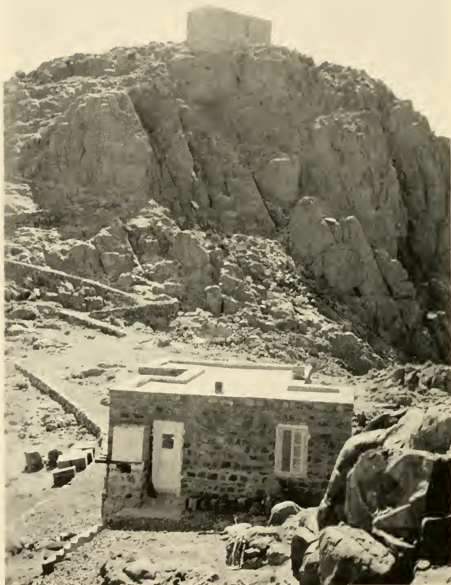
VIEW SHOWING THE WEST AND NORTH SIDES OF THE OBSERVATORY AND THE DWELLING. MOUNT ST. KATHERINE
