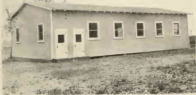
1. Shop erected at Roswell, N. Mex., in September 1930.
