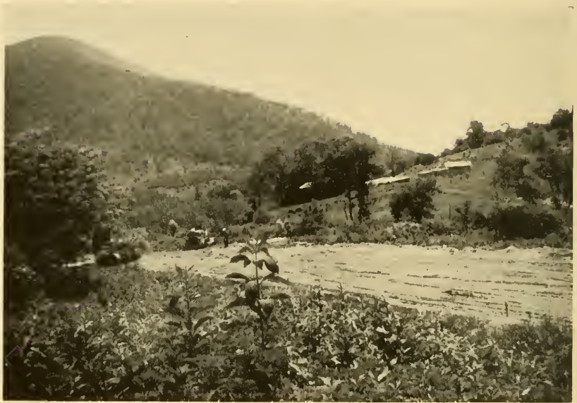
1. The site, partly graded, showing Flat Top in the distance.
