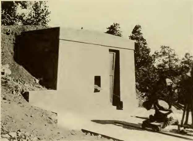
FIG. 32.—Concrete observing tunnel at Table Mountain, California.
