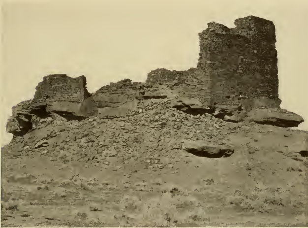
FIG. 103.—Wukoki (near Wupatki Monument). It is hoped that Wukoki may later be included in the Monument.
