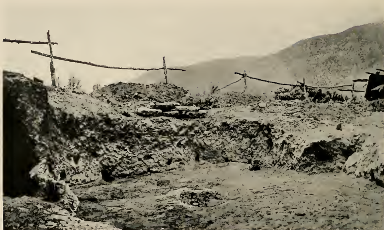
Kiva III from the southwest; the two central fireplaces appear indistinctly in the foreground; numerous squirrel burrows pierce the walls.
