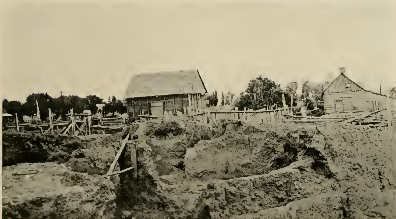
Kiva I from the north wall of Room 2, shown at the lower right; Fireplace B at the left of the braces which support the east wall of the ceremonial room.
