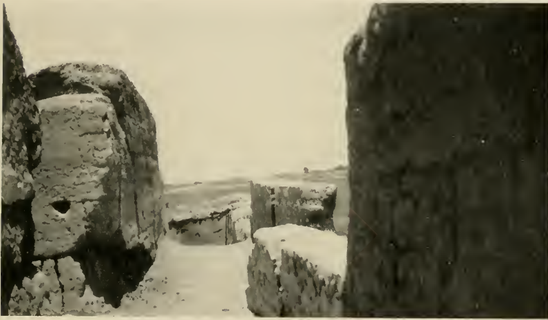
FIG. 75.—Corridor of the small palace at Pando. A dwelling of present inhabitants in the background of the picture.
