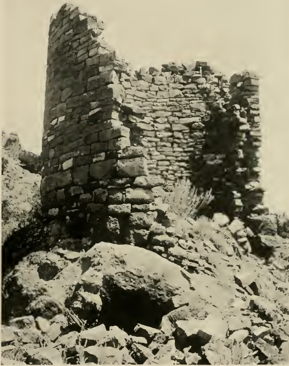
FIG. 79.—D-shaped tower, McLean Basin, Utah. Photograph by J. Walter Fewkes.
