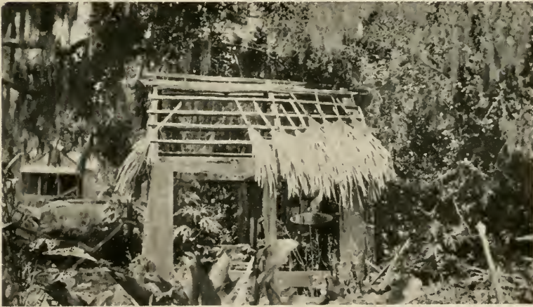
FIG. 105.—Method of constructing a palmetto roof. Indian house at Point au Chien, Terre Bonne, La.
