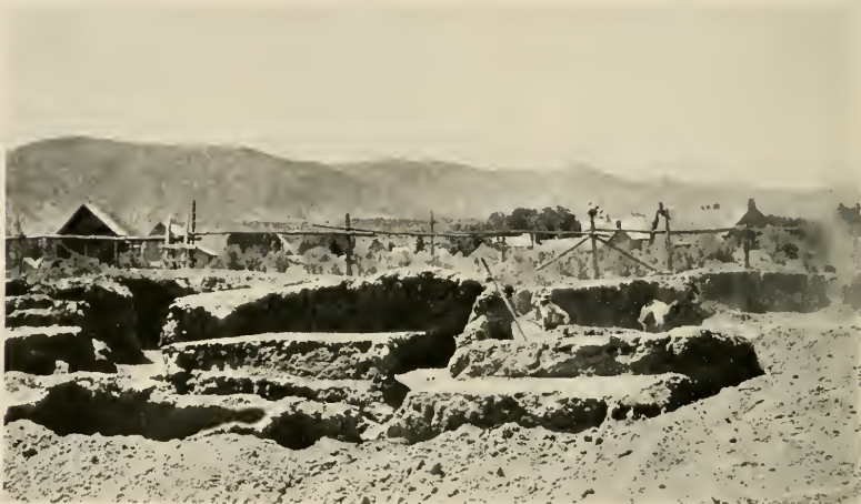
FIG. 85.—In the foreground may be seen the walls of three superposed dwellings in the great mound at Paragonah. The ancient builders apparently leveled the walls of a house which had collapsed and, without removing the wreckage, built a new structure above the remains of the former.
