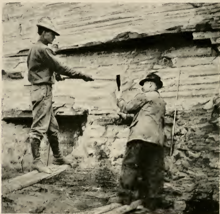
FIG. 3.—Undercutting by blasting in order to get at the fossil-bearing bed of rock in the famous Burgess Pass quarry. William Oke and Alex. Mitton drilling, while standing on poles high above the floor of the quarry. Photograph by Walcott, 1917.
