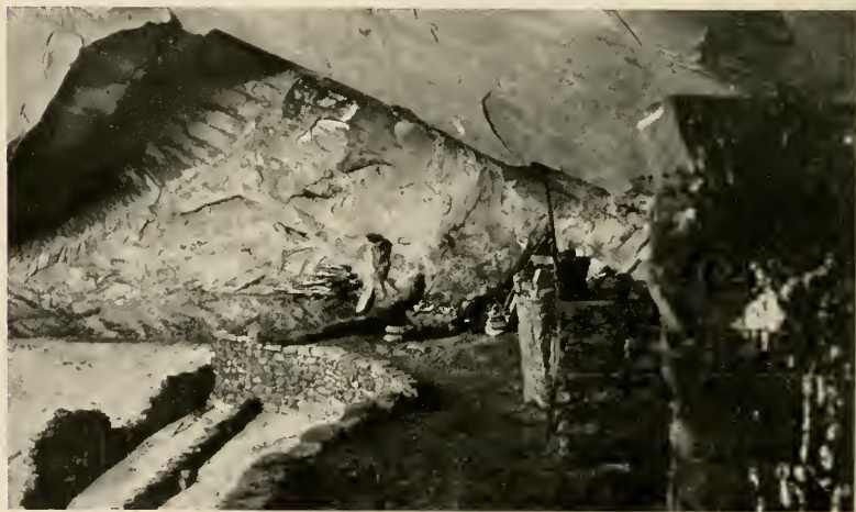
FIG. 82.—Approximately the same view, after the work of excavation and repair. Note the restored retaining wall in the middle foreground. It forms a walk or platform in front of a row of houses whose outer walls were of wattle construction.
