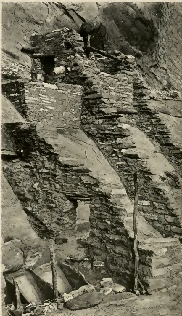
FIG. 78.—Restored walls and mealing room, on the sharply sloping cave floor at Betatakin. The original of the wall at the extreme right collapsed after a heavy fall of snow; the front wall of the house at the top fell during a particularly severe thunderstorm, while workmen were engaged below. The three parallel walls are restorations.
