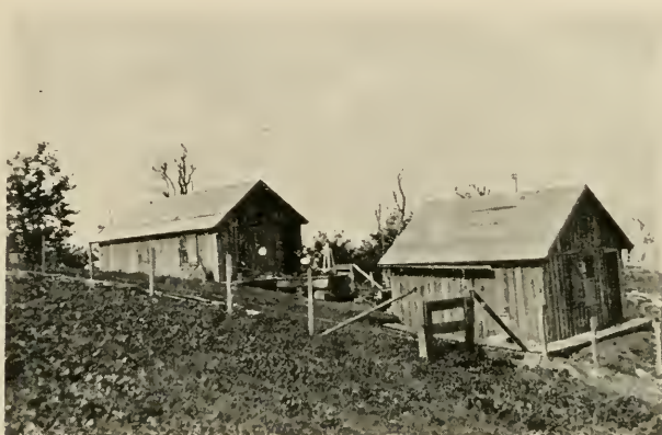
FIG. 25.—Observatory and cook-house, Hump Mountain, N. C.
