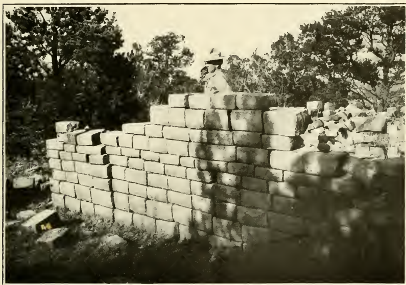
FIG. 54.—Character of masonry shown in one of the house-groups of the compound. Note the failure of the builders to “break” the joints and the consequent weakening of an otherwise excellent wall. The face of the stones is pecked to smoothness and all the stones are artificially squared. Photograph by Nusbaum.
