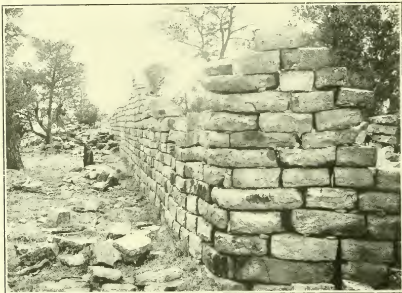
FIG. 55.—Stone outer wall of a defensive structure near the mesa rim. This wall is about 132 feet long in the clear, and is pierced only by small loop-holes. Photograph by Nusbaum.
