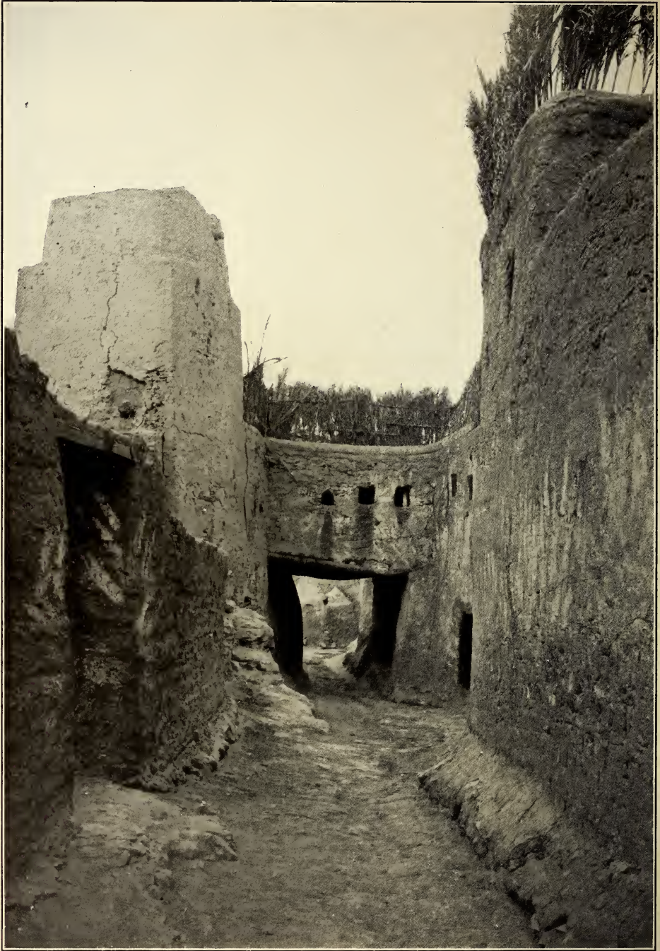
KHARGA OASIS : A STREET IN KHARGA VILLAGE
