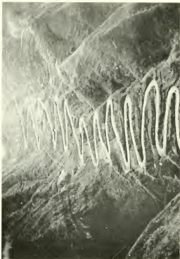
2. A motor road on a steep hillside between Yunmaiti and Chungking, with 24 hairpin turns.
