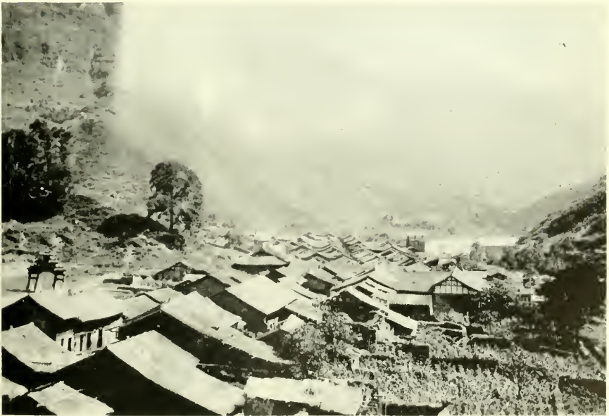
2. The Chinese town of Mu-p'ing, in the highlands of Sikang, typical of thousands of Chinese towns and villages before the streets were widened. The houses and stores have tile roofs.
