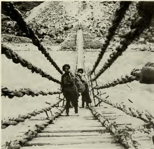
Upper , Chi'ang woman and girl wearing woven belts. Lower , The rope bridge consisting of bamboo cables and boards across the Min River at So-ch'iao. The weight of this bridge sometimes breaks the bamboo cables.
