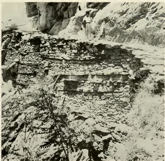
Upper , A cobalt bridge near Wei-kuan in the Ch'iang region. Lower , Ch'iang road built over a cliff.
