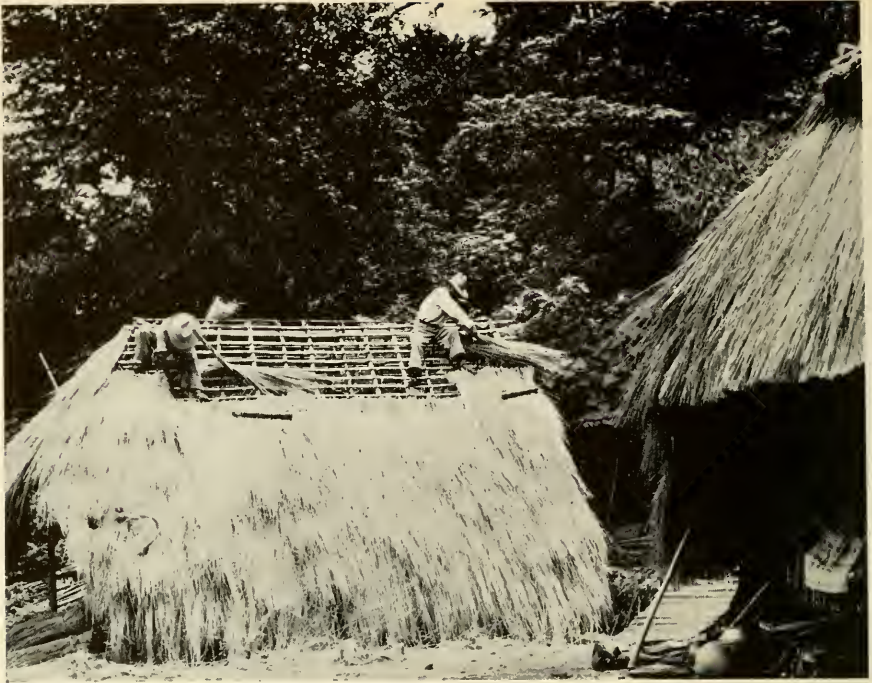
1. Construction of native dwelling (ranchito). Usually the roof must be replaced every 5 years. Neighbors often cooperate in accomplishing this task.
