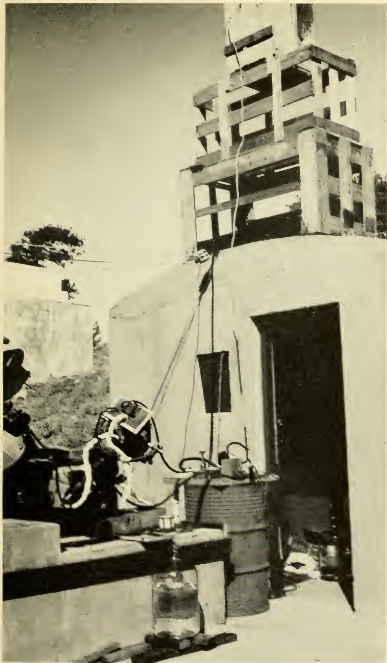
STANDARD WATER-FLOW PYRHELIOMETER AS MOUNTED AT TABLE MOUNTAIN, CALIF.
