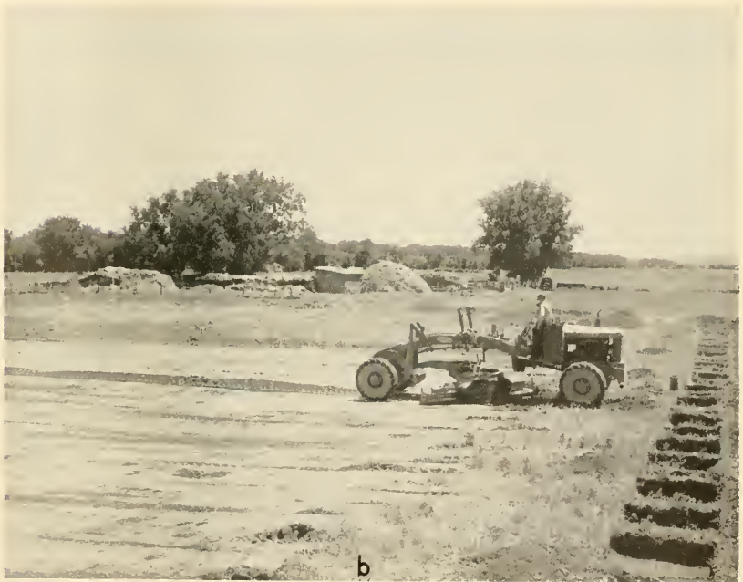
a , Site of Fort Pierre II (39ST217) prior to excavation; cellar pit right center; farm buildings rear. b , Blading operations; exploratory trenches (right) mark west stockade line.
