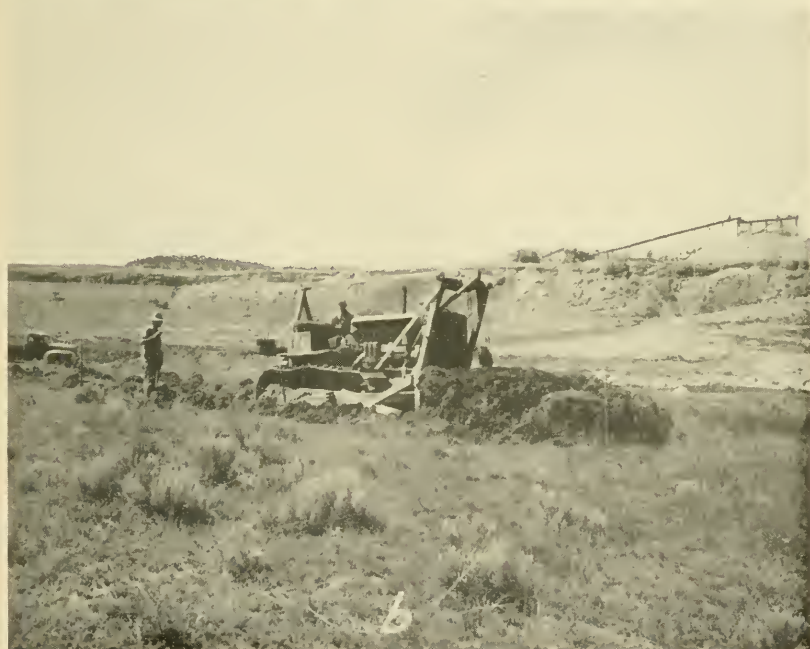
a , Aerial view of Angostura Dam (center foreground) and part of reservoir area beyond, Angostura Reservoir, S. Dak. Circles indicate some of the archeological sites within the future pool area. (Neg. 39FA00-20.) b , Bulldozer of Utah Construction Company removing sod at start of archeological tests at 39FA10, Angostura Reservoir, S. Dak. Part of construction area visible in background. (Neg. 39FA10-2.)
