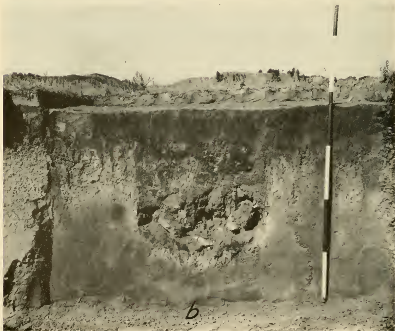
a , Workmen excavating stone-lined fireplace basin at 39FA9, Angostura Reservoir, S. Dak. (Neg. 39FA9-15.) b , Deep hearth or roasting pit containing burnt stones and sooty soil, exposed during road construction; Angostura Reservoir, S. Dak. (Neg. 39FA68-2.)
