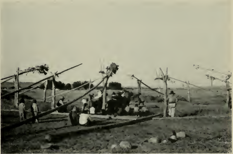
Upper: How the rafters are raised. Only one set of joined poles is being used here. Lower: Getting ready to lift the center pole. The tips of the rafters have been placed in the forks of the side posts; the east-running rafter is lying in the foreground.
