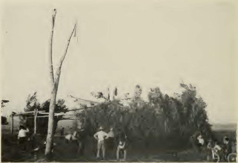
Upper: Men putting up the side roof poles, July 3, 1937, 6:50 p. m. Lower: The brush wall being finished, July 3, 1937, 7:30 p. m.
