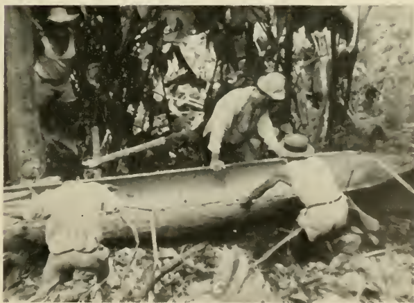
a, Working on canoe before hauling. b, Hand adz at work on interior of canoe. c, Preparation for hauling canoe.
