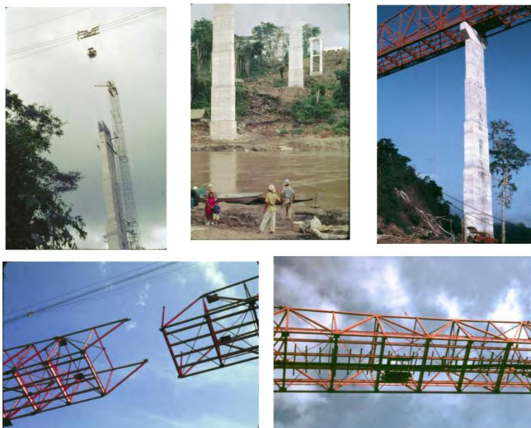
Photos 5: The Bayano Bridge under construction in December, 1973. Source: Bob Webb, 2008
