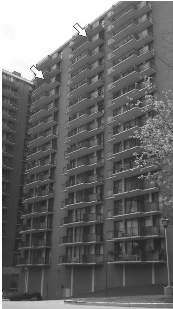
Fig. 1. Arrows mark the location of hummingbird feeders on the balconies of a high-rise apartment building in College Park, Maryland. The highest feeder was 43 m above ground level.
