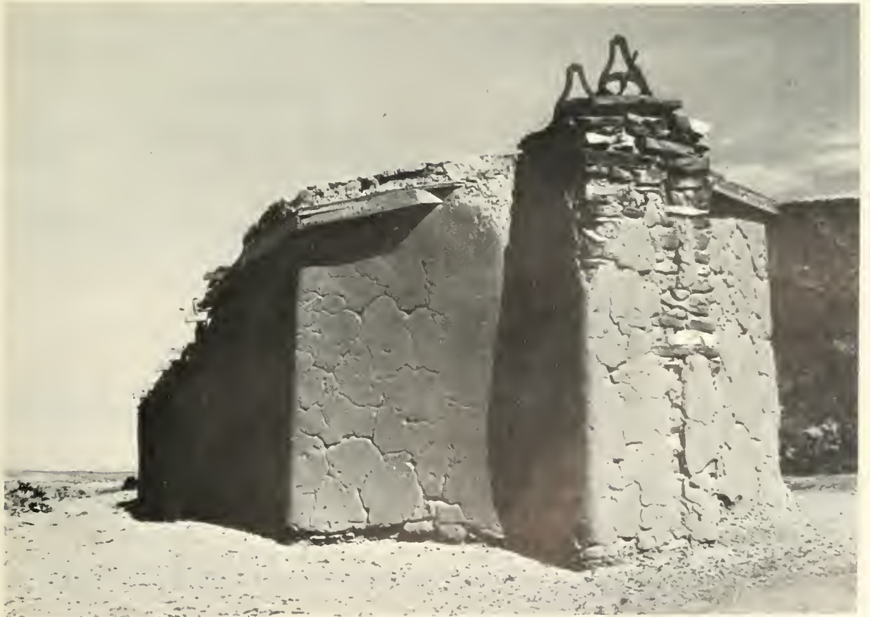
FIGURE 8. Northwest view of east morada , showing limestone slab bell tower on contracted west end.
