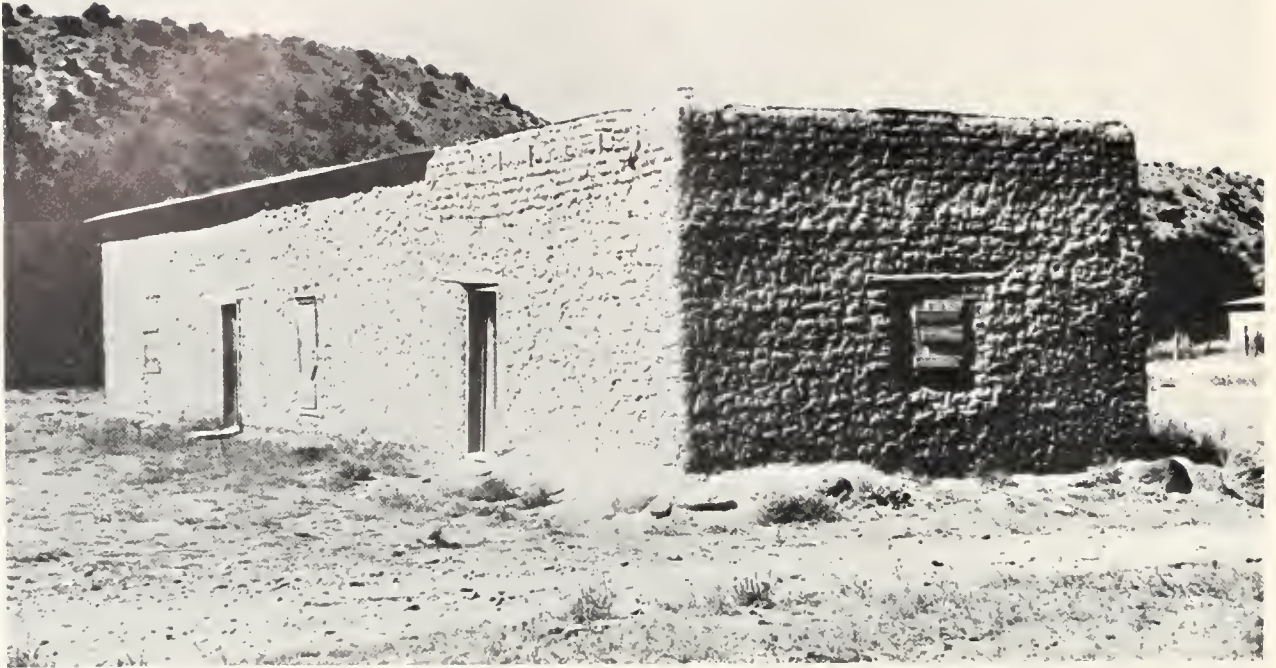
FIGURE 5. SOUTH Morada . SIZE: 24.02 meters long, 5.41 wide, 3.51 high. DATE: About 1900. LOCATION: 400 meters south of Santo Tomás Church in main plaza; seen from southeast corner. MANUFACTURE: Adobe bricks on stone foundation; wood door and window frames.
