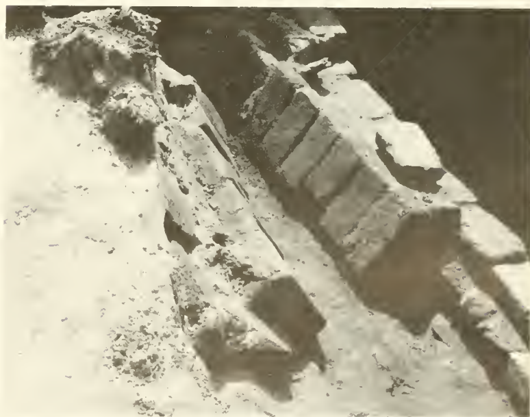
Figure 5.—DETAIL OF COLLAPSED BRICKS in the underhearth. (Photo courtesy of E. DeHardit.)
