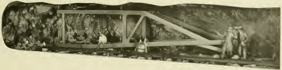
Figure 3.—HOOSAC TUNNEL. WORKING OF LATER STAGES with Burleigh pneumatic drills mounted on carriages. The bottom heading is being drilled in preparation for blasting out with nitroglycerine. MITH model— \frac{1}{2} " scale. (Smithsonian photo 49260-M.)
