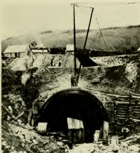
Figure 14.—WEST PORTAL OF HOOSAC TUNNEL before completion, 1868, showing six rings of lining brick.
