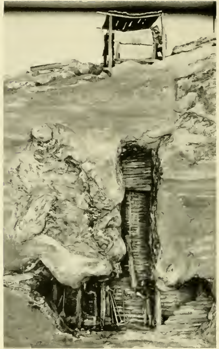
Figure 17.—SOFT-GROUND TUNNELING. The support of walls and roof of mine shaft by simple timbering; 16th century. MHT model— \frac{3}{4} " scale. (Smithsonian photo 49260-J.)
