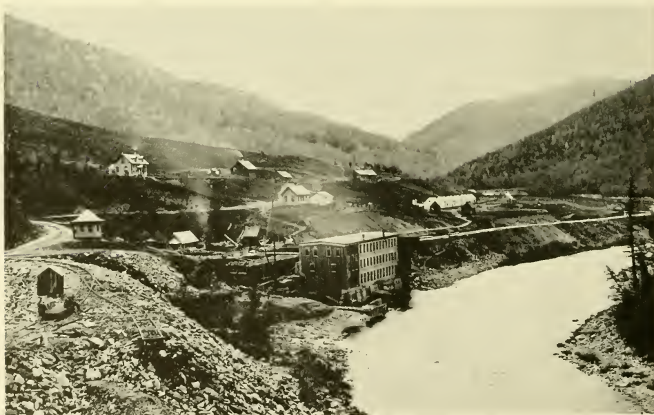
Figure 13.—HOOSAC TUNNEL. AIR-COMPRESSOR BUILDING on Hoosic River near North Adams. The compressors were driven partially by waterpower, derived from the river. ( Photo courtesy of State Library, Commonwealth of Massachusetts. )
