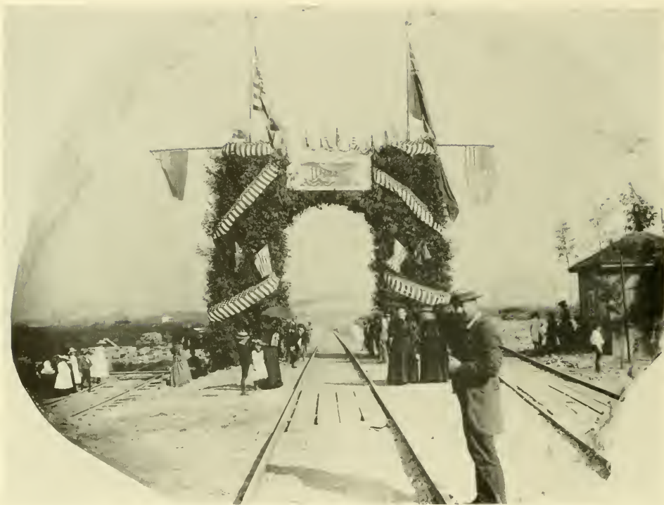
Figure 44.—OPENING OF THE ST. CLAIR TUNNEL, 1891. (Photo courtesy of Detroit Library, Burton Historical Collection.)
