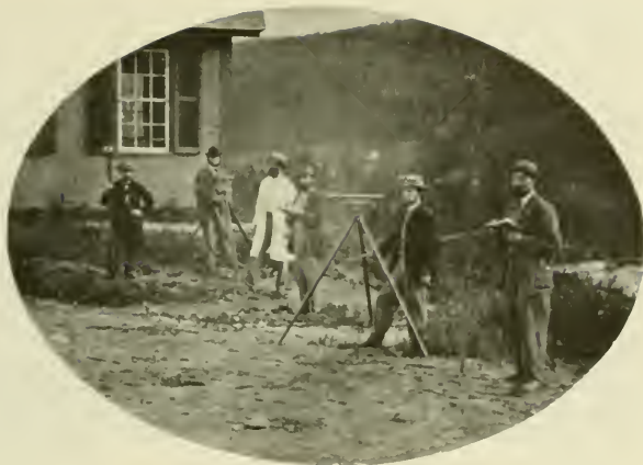
Figure 11.—HOOSAC TUNNEL survey crew at engineering office. The highest accuracy of the aboveground and underground survey work was required to insure proper vertical and horizontal alignment and meeting of the several separately driven sections. (Photo courtesy of State Library, Commonwealth of Massachusetts.)
