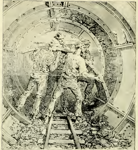
LINING THE CONCRETS.
