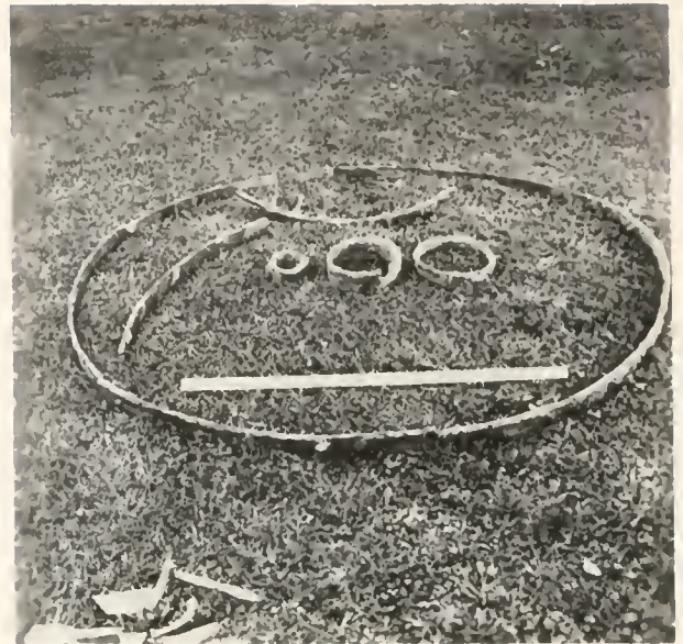
Figure 3.— SIX STRAKES ARRANGED IN A CIRCLE, as they would encompass a 12-spoke wheel. In the center are two extra stakes, two hub bands, and a hub boxing (the smaller ring).
