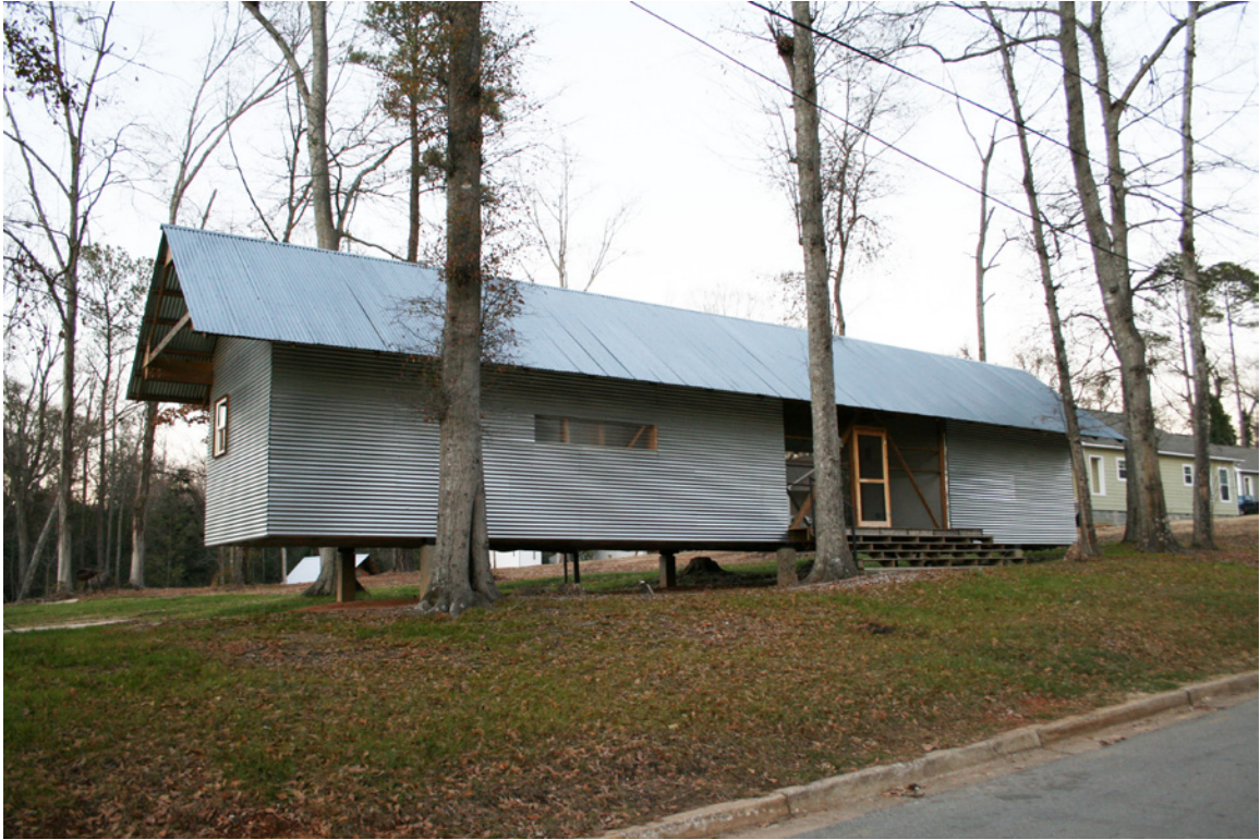
Detail of 20K House in the North Ward subdivision, by the Rural Studio, 2008. Photo by the Author, 2011.
