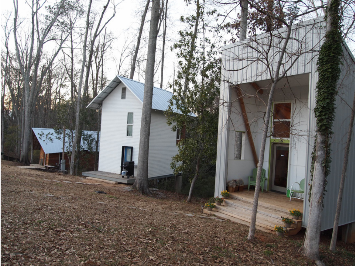
20K Houses in the North Ward subdivision, by the Rural Studio, 2008. Photos by the Author, 2011.
