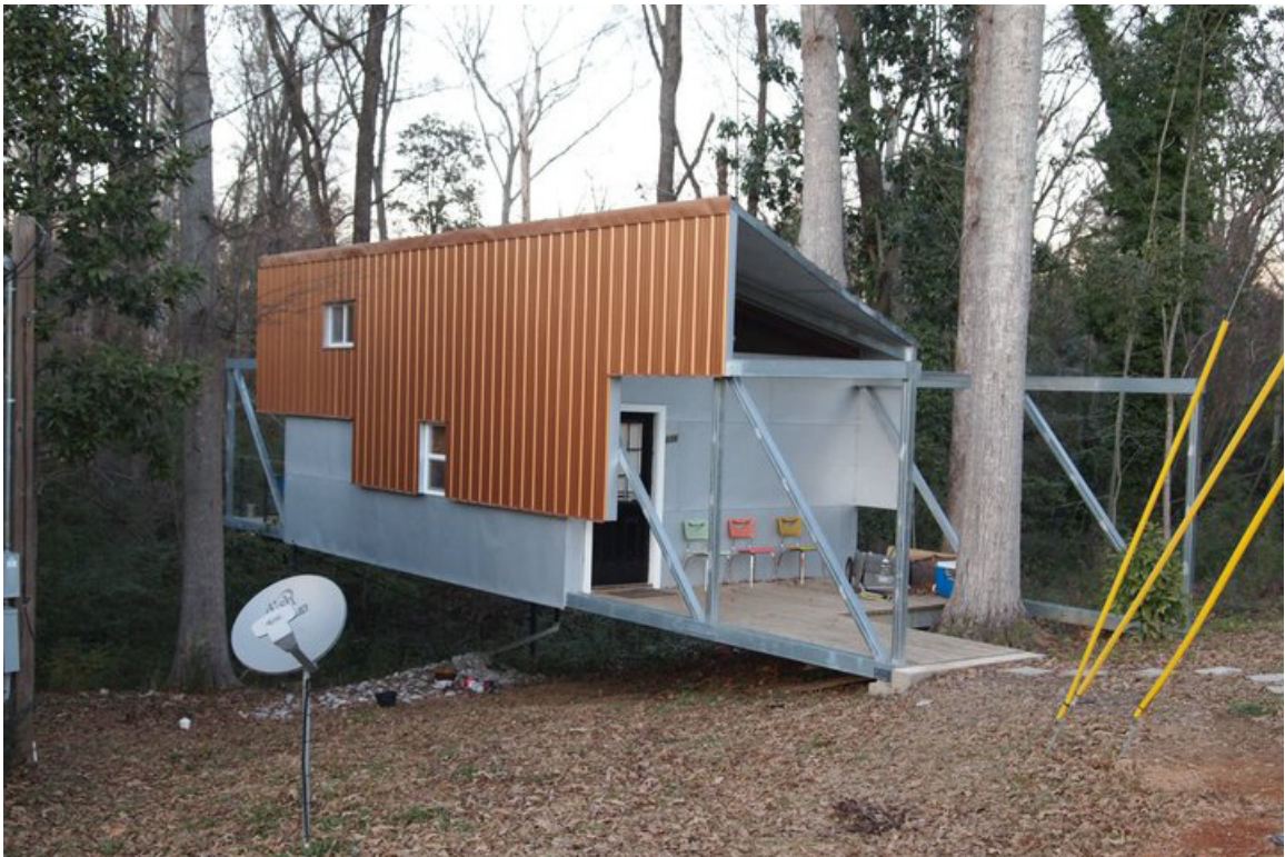
Detail of 20K House in the North Ward subdivision, by the Rural Studio, 2008. Photo by the Author, 2011.
