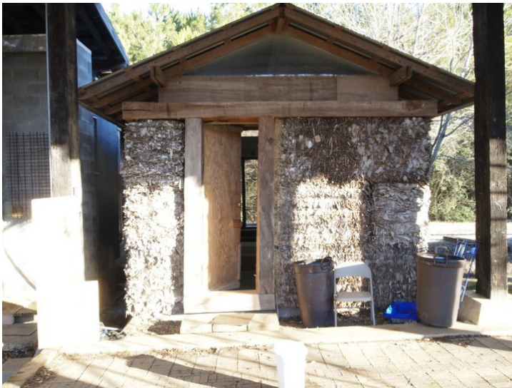
Details of housing pods for Rural Studio students using experimental building materials, by the Rural Studio, 2000. Photos by the author, 2011.
