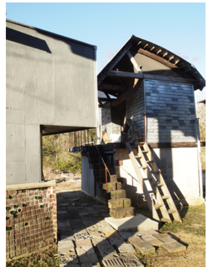
Details of housing pods for Rural Studio students using experimental building materials, by the Rural Studio, 2000. Photos by the author, 2011.
