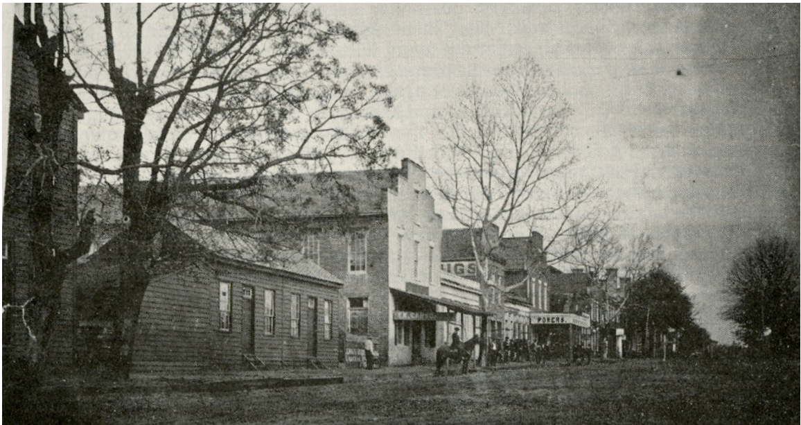
View of south side of Main Street in Greensboro (1873). From: Curb, Randall, and Willie Jean Arrington. Historic Hale County . Greensboro, Alabama: Greensboro Watchman, 1989.
