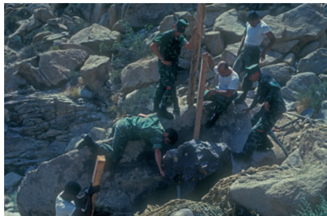
Fig. 4. Riggers from the First Marine Division Landing Support Co. at Camp Pendleton use jacks and timber to maneuver the meteorite so that a double thickness of cargo net can be placed under it and it can be airlifted by helicopter from the mountains. The photo was taken by Joe Goodwin at 3:00 p.m. on June 16, 1977.
