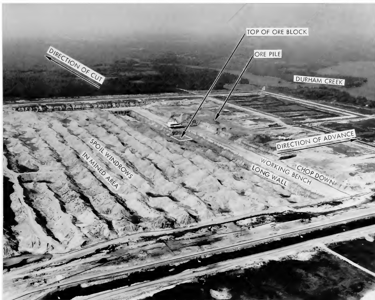
FIGURE 3.—Oblique aerial view of mine area, 1972, looking southward. At this writing, mining has reached Durham Creek, turned southward, and now eastward, and the spoil area shown here, a rich source of fossils, has been reclaimed. Courtesy of Texasgulf Inc.
