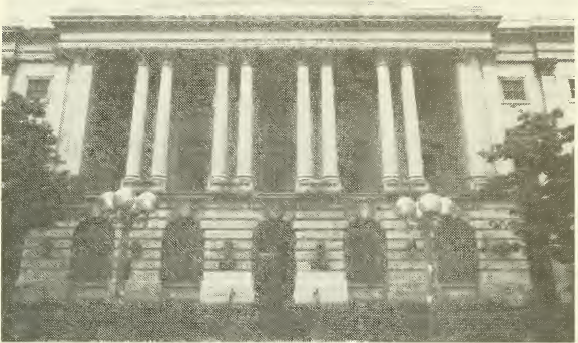
General Post Office Building, view of the F Street Entrance.
