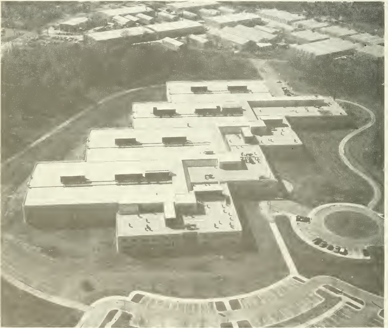
The zigzag design of the Museum Support Center (dedicated in May 1983) creates maximum adjacency between the four-pod, loft-like storage area and the separate, two-story office/laboratory complex; it also makes the building easily expandable.
