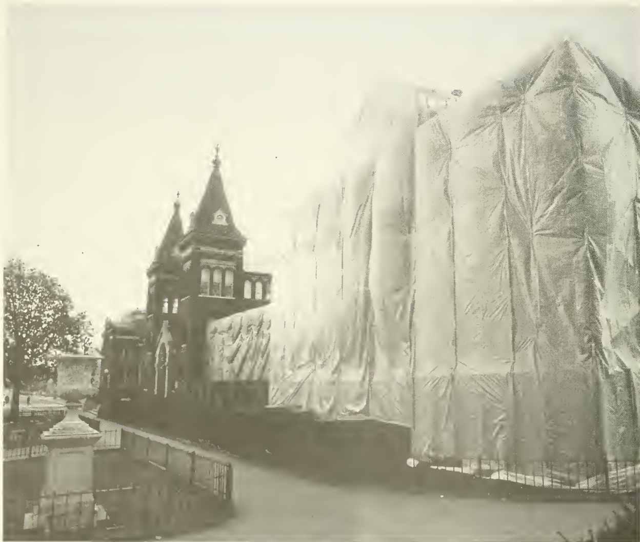
First phase of roof replacement for the Arts and Industries Building, completed in FY 1983.
