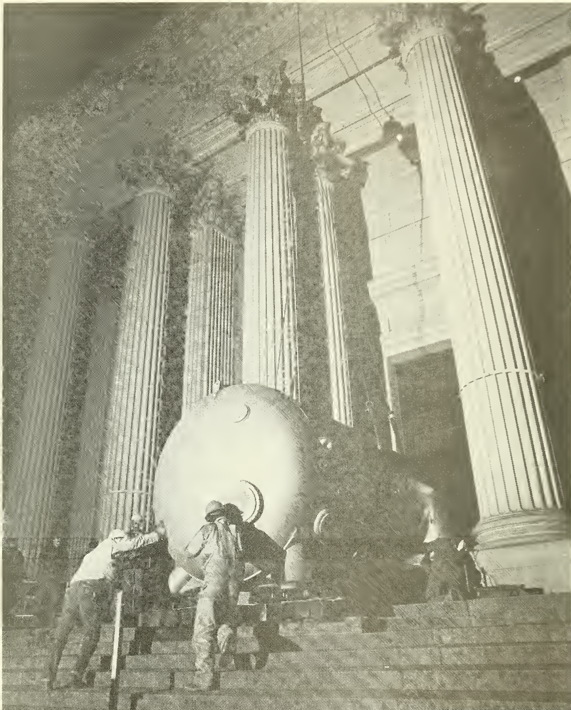
Workmen move Hydrolab into the National Museum of Natural History. The 18-foot long, 8-foot high tanklike underwater research habitat is the largest manmade object ever transported to the Museum for an exhibition. It is on long-term loan from the National Oceanic and Atmospheric Administration. Photo by Chip Clark.
