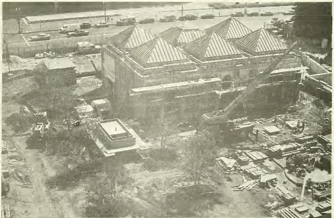
Quadrangle construction nears completion. Upper photo shows African pavilion copper roofing and skylight, with fountain construction in the foreground. Lower photo shows granite installation on Sackler pavilion north facade and completion of copper roofing. Photo by Frank Gilmore.
