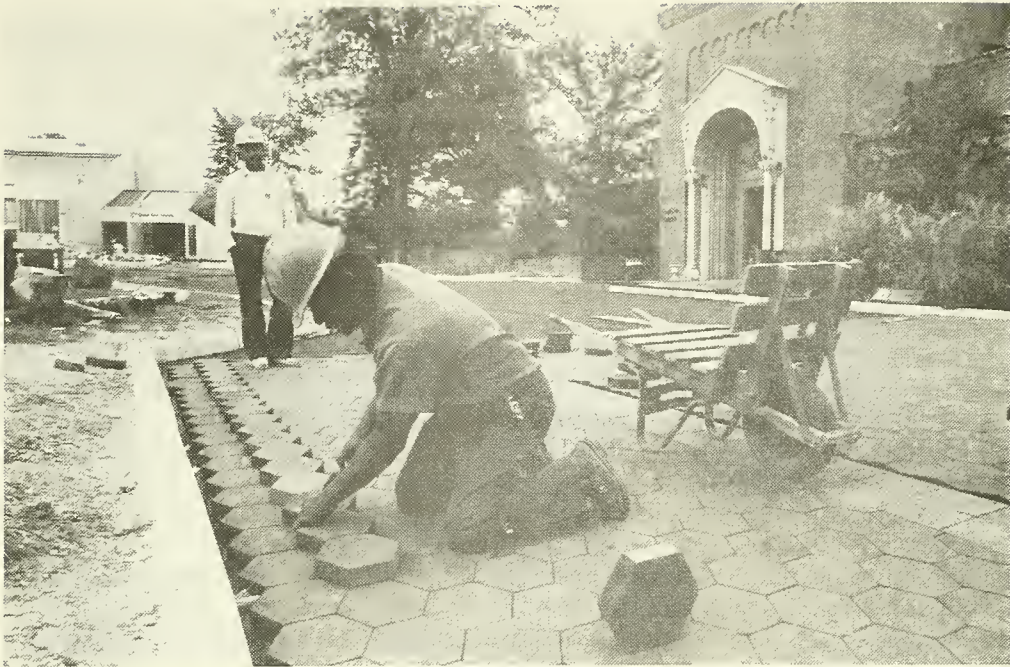
Workman lays hexagonal pavers along Olmsted Walk, the main pedestrian path through the National Zoo. The renovation of this walk should be complete by 1989, in time for the Zoo's centennial. Photo by Jessie Cohen.
