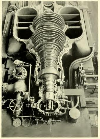
Steam turbine, Parsons type. Top view. Capacity 30,000 kilowatt, 1,800 r.p.m. Courtesy of the Allis-Chalmers Manufacturing Company
