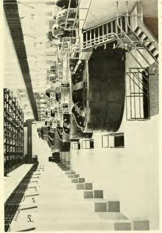
Niagara Falls. Interior of Schoelkopf Station. Three 37,500 h.p. generators in the foreground, three of 70,000 h.p. at the rear. Courtesy of the Niagara Falls Power Company
