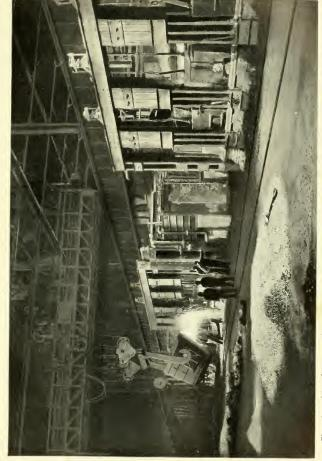
Charging side of an open-hearth furnace steel plant. Courtesy of the United States Steel Corporation
