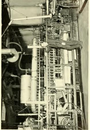
Incandescent light bulb machine. Blows 400,000 bulbs per day. Courtesy of the Corning Glass Works
