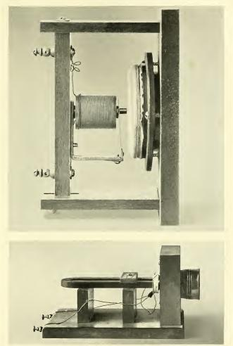
Upper: Bell's original telephone. Lower: Bell's original box telephone
