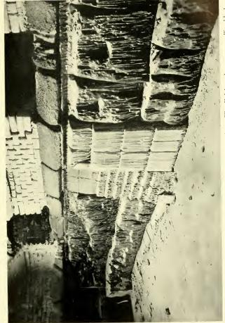
Differences between refractories in withstanding hot glass action. The Fulcher electrocast mullite blocks occupy the center of the furnace wall. Courtesy of the Corning Glass Works
