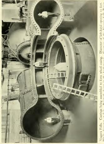
Niagara Falls. Castings being assembled to form wheel casing. Whole diameter 47 feet. Penstock shown in the background. Company
