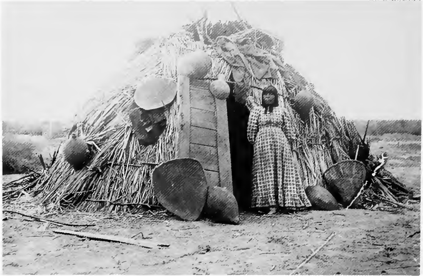
Figure 12. Cattail house with wooden door, Freeman ranch, Stillwater, Nevada, ca. 1890. Photograph by Mary Freeman. Courtesy of Special Collections Department, Getchell Library, University of Nevada, Reno.
