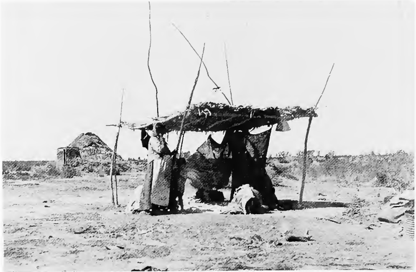
Figure 58. Four-post shade roofed with cattail mats. Photograph by Mary Freeman, Stillwater, Nevada, ca. 1900. Courtesy of Special Collections Department, Getchell Library, University of Nevada, Reno.
