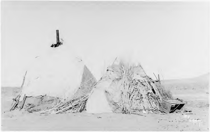
Figure 56. Cattail houses with postcontact additions of cloth, central stove. Photograph by Rolly Ham, ca. 1902, near Fallon, Nevada. Courtesy of Special Collections Department, Getchell Library, University of Nevada, Reno.
