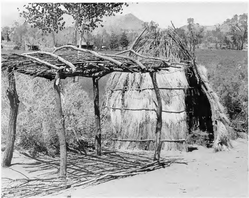
Figure 61. Dome-shaped Northern Paiute house covered with Great Basin wild rye, Pyramid Lake, Nevada. Willow and pole-covered shade to the left. Made by Mabel Wright, ca. 1965. Photograph by M.M. Wheat. Courtesy of Special Collections Department, Getchell Library, University of Nevada, Reno.
