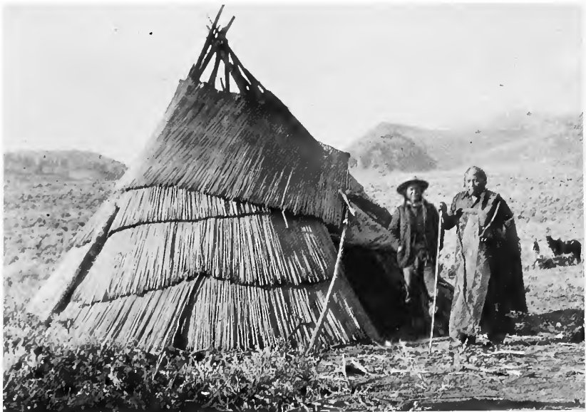
Figure 60. Conical tipi-like structure covered with sewn tule mats. Northern Paiute chief Ocheo is to the right. Photographer, date, and place unknown, but prior to 1906 and probably in southeastern Oregon. Courtesy of National Anthropological Archives (Neg. No. 1658), Smithsonian Institution.
