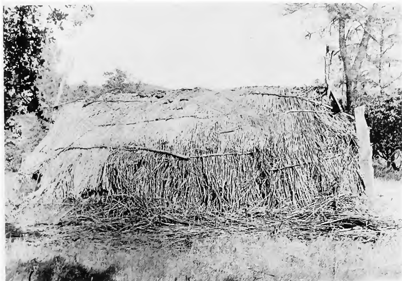
Figure 62. Deserted Pomo tule house, Clear Lake, California, 1906. Photograph by S.A. Barrett. Courtesy of Lowie Museum of Anthropology (Cat. No. 15-2769), University of California, Berkeley.
