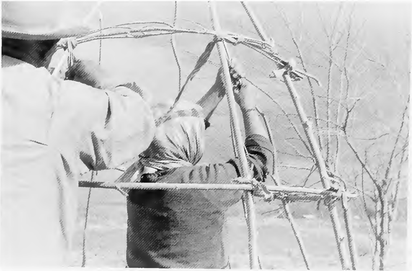
Figure 52. Jimmy George and unidentified woman securing horizontal willow rings to framework of a cattail house, ca. 1958. Photograph by M.M. Wheat. Courtesy of Special Collections Department, Getchell Library, University of Nevada, Reno.
