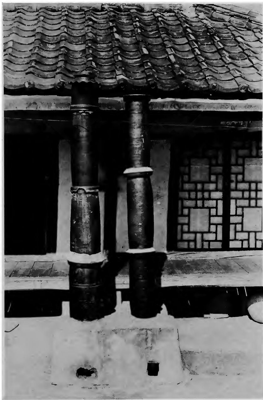
Figure 27. House near Kyongju, N. Kyongsang Province, with ceramic tile roof and chimney pipes. The latter (kul tuk) vent smoke and soot from the dwelling's kitchen hearth. (Photo by Ralph Rinzler, 1972.)
