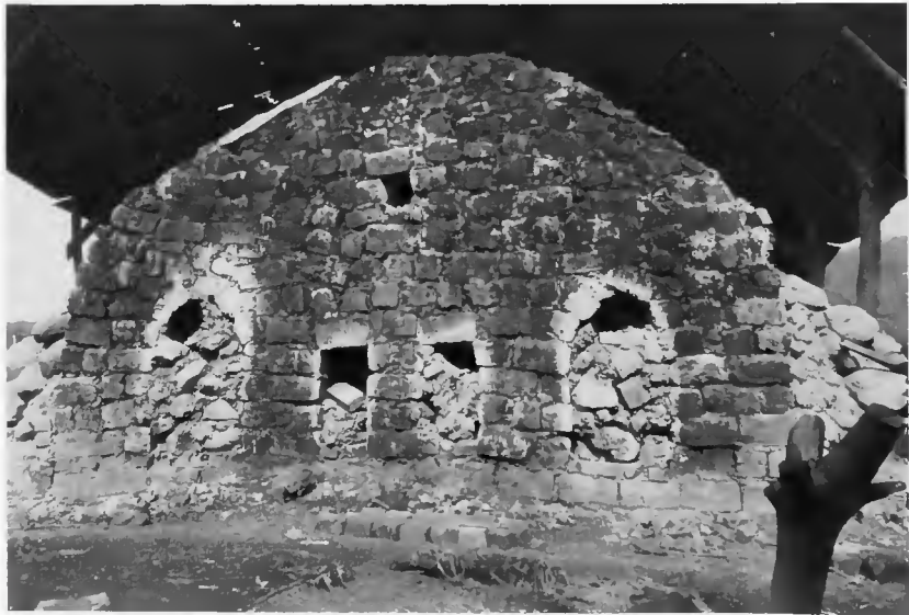
Figure 39. Chimneyless upper end of kiln in Figure 38 showing flue openings. Fuel drops line both sides of kiln at approximately 40-cm intervals. (Photo by Ralph Rinzler, 1971.)
