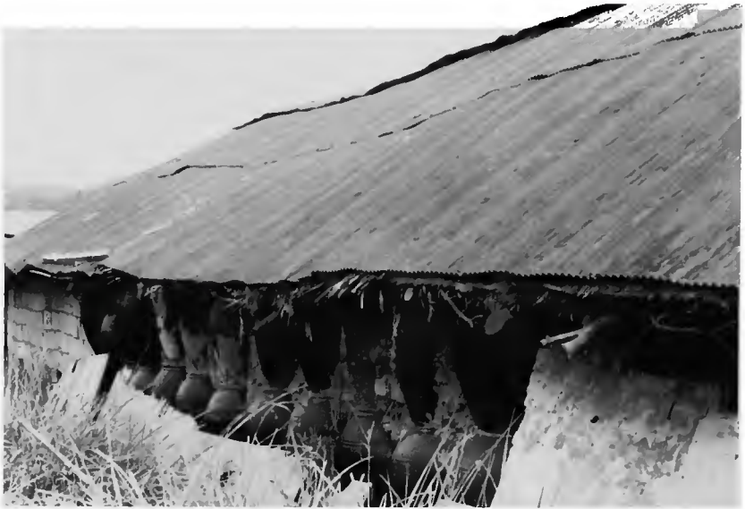
Figure 105. Damaged storage jars used as wall fill at Mangyang village. (Photo by Ralph Rinzler, 1981.)
