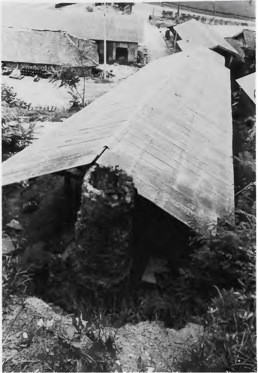
Figure 88. Upper end of second noborigama at Kūnnam Factory. Chimney stacks are a distinctive feature of most chamber kilns. (Photo by Ralph Rinzler, 1981.)
