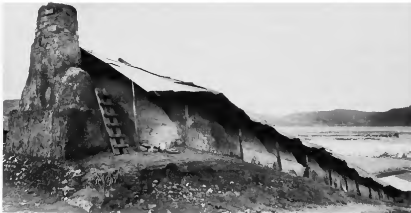
Figure 107. Upper end of steeply sloping chamber kiln (kaeryanggul) at Mangyang village, showing distinctive chimney. Entry to chambers along right side. (Photo by Ralph Rinzler, 1981.)
