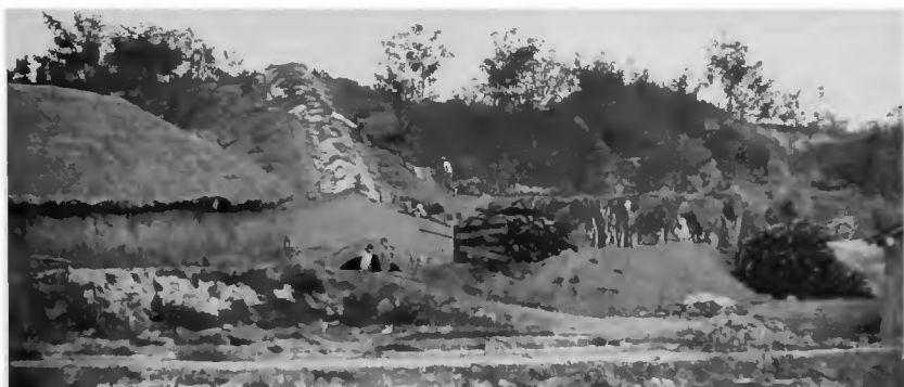
Figure 73. Cannon kiln at Kaya village. This small, uncovered structure, vented through five flues at the upper end, seems to be the archetype for Korean onggi kilns before ca. 1970. (Photo by Ralph Rinzler, 1972.)
