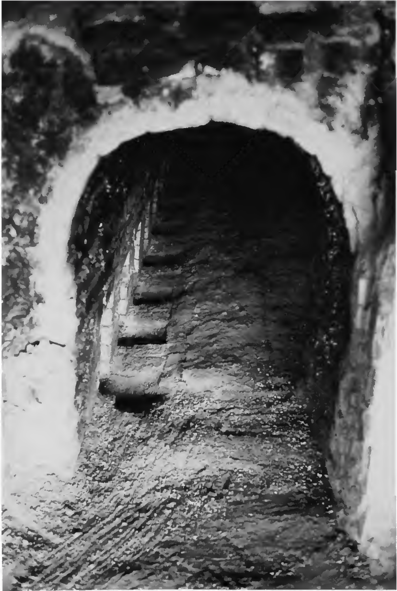
Figure 50. Floor-level vents in wall dividing chambers. (Photo by Ralph Rinzler, 1981.)
