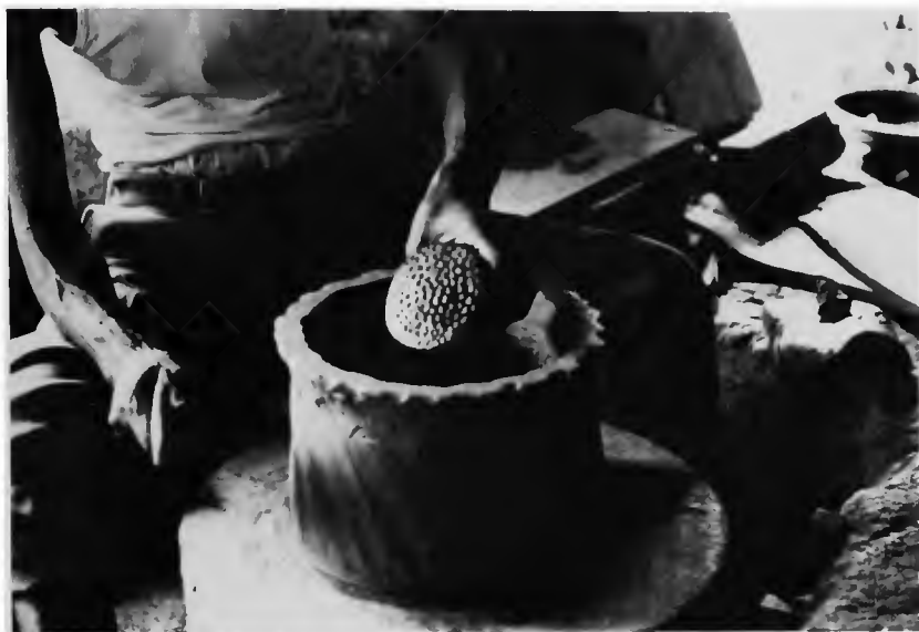
Figure 92f. Cylinder wall contoured with paddle (surae) and anvil (ch'ōmak).
