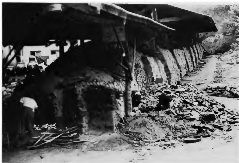
Figure 86. Chamber kiln (norigama) at Kūnnam Factory. Each of 12 chambers (entry on opposite side) is approximately 3.7 meters deep. (Photo by Ralph Rinzler, 1981.)
