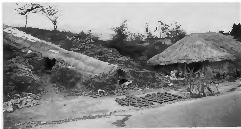
Figure 93. Onggi factory at Wōnbang village, S. Chōlla Province. The narrow cannon kiln, measuring 27 meters in length, was fired over nine days (10 during damp weather), using pine roots for fuel. Both it and the adjacent work building had been razed by 1981. (Photo by Ralph Rinzler, 1972.)
