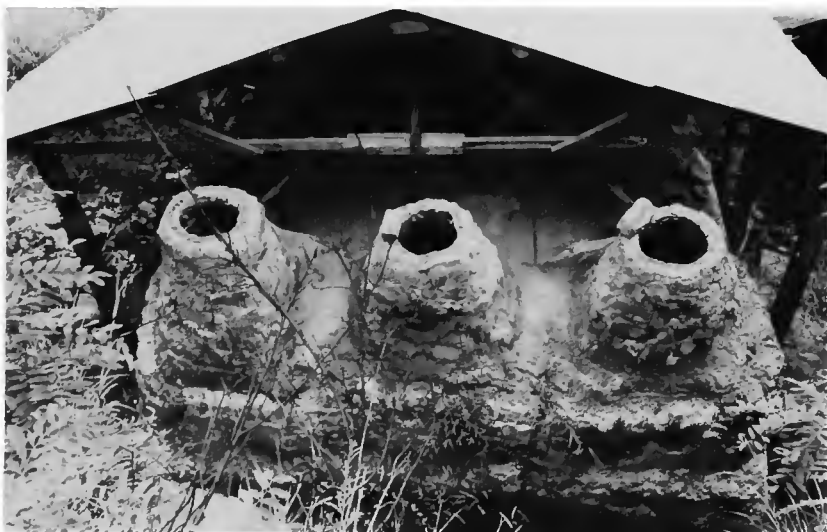
Figure 87. Three-chimney configuration of kiln in Figure 86. Each chimney is 2.6 m high; base is 5.0 m wide. (Photo by Ralph Rinzler, 1981.)
