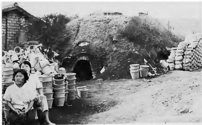
Figure 31. Beehive-shaped kiln for firing unglazed flowerpots, Puch'ŏn, Kyŏnggi Province. (Photo by Ralph Rinzler, 1971.)
