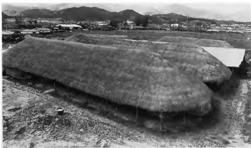
Figure 42. Ware storage shelters and workroom (small structure in rear) at Sōnggwang Factory, Kap'yōng, Kyōnggi Province. The thatched roofs on all three buildings were intact 10 years after this photo was taken but had been covered over with sheet metal, the result of a rural improvement campaign. (Photo by Ralph Rinzler, 1971.)
