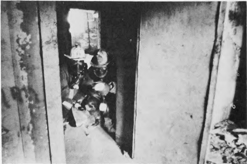
Figure 15. With masks in place, the engine company officer (white hat) and the line man begin to advance the hose line into the fire room.
