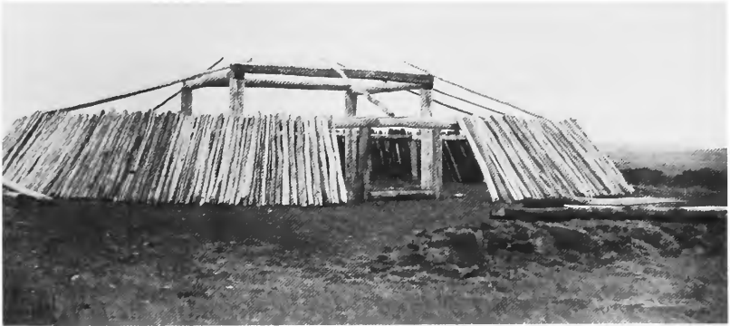
Figure 43. Arikara dance lodge under construction. The four central posts were a structural feature retained in some Ojibwa Drum Dance halls, such as that at Lac Vieux Desert and the hall (fig. 42) at Lac du Flambeau. (Photo courtesy American Museum of Natural History, neg. no. 15981.)
