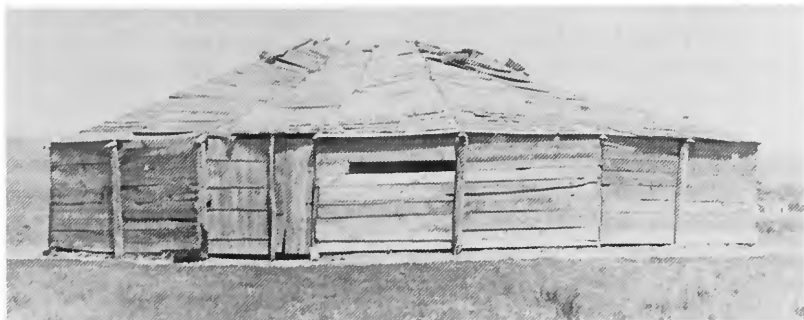
Figure 39. Another Siouan dance hall of the same period built of board and made to approximate a circle. Nearly all such halls shared the peaked roof. (Photographer unknown, courtesy NAA, neg. no. 53396.)
