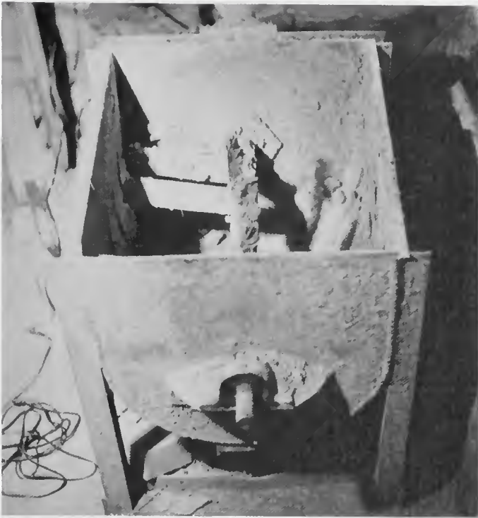
Figure 15. Lanier's electric mud mill. (Photo by Robert Sayers, 1979.)
