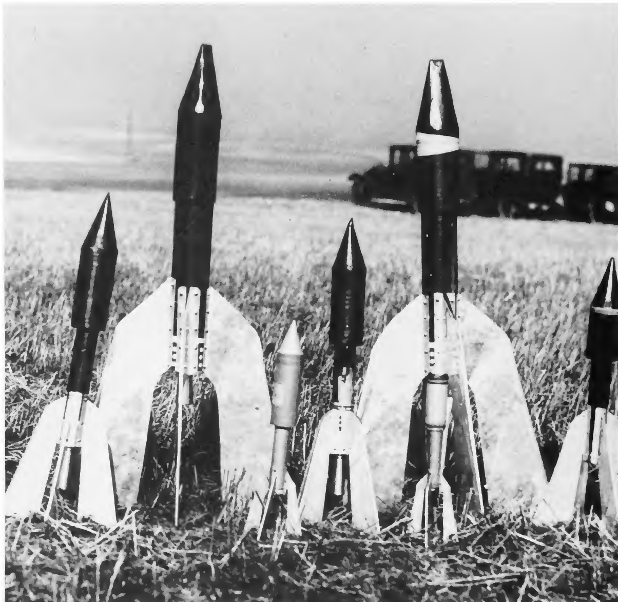
FIGURE 1.—Some of the solid propellant rockets developed by Ludvík Očenášek.
