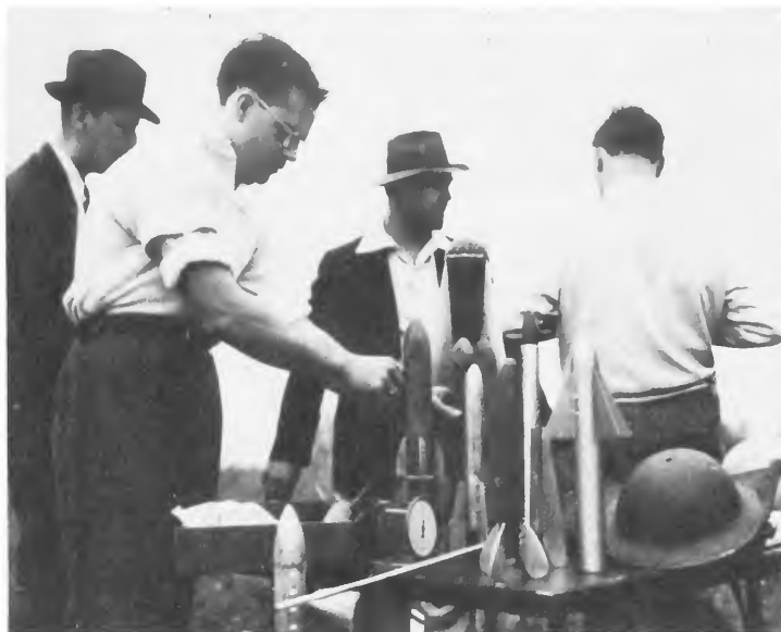
FIGURE 13.—H. F. Pierce, with solid-fuel rockets of various designs tested by the Committee to determine the best aerodynamic shape and other characteristics of high-altitude rockets. These tests took place principally at a site near Pawling, New York, where this picture was taken in 1935, during one of the earliest series. These rockets and those in Figure 14, were constructed by various members of the Experimental Committee and were powered by commercial 4-pound and 6-pound skyrocket motors.
