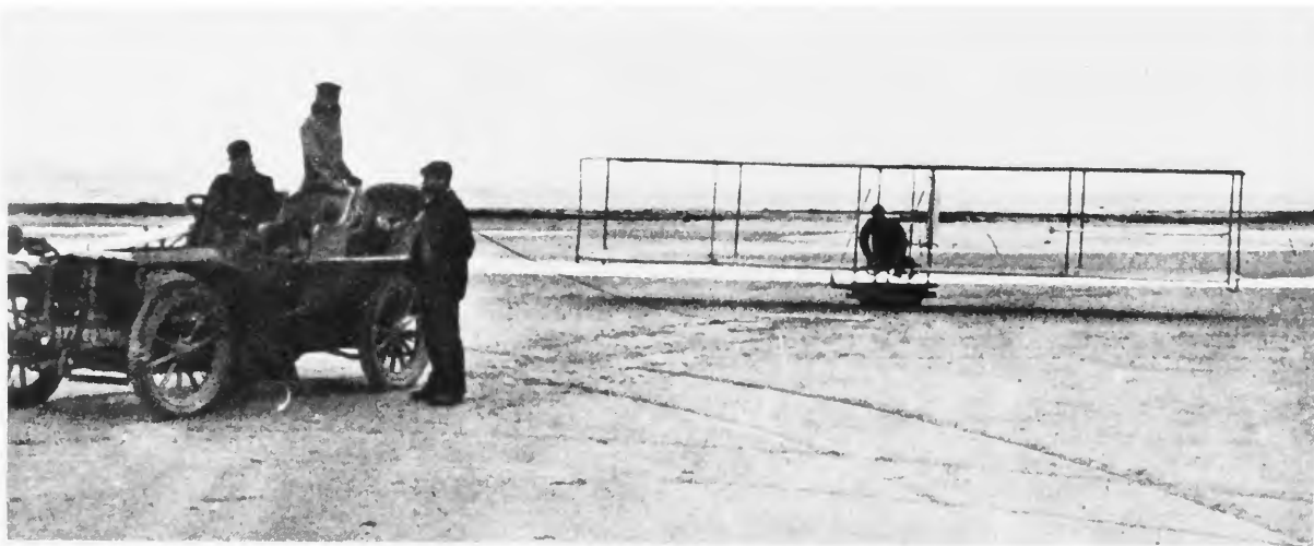
FIGURE 2.—Glider designed and constructed by Robert Esnault-Pelterie prior to towing test by auto, 1904.
