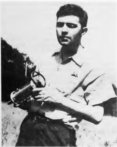
FIGURE 17.—James H. Wyld and a model of his liquid-propellant regenerative rocket motor at Midvale, New Jersey, on 8 June 1941, just prior to a successful test of the motor. In subsequent tests on the ARS No. 3 proving stand, which provided larger fuel capacity and hence longer runs, the Wyld motor did not burn out, and it delivered a thrust of somewhat more than 90 pounds and a jet velocity of well over 6,000 feet per second.
