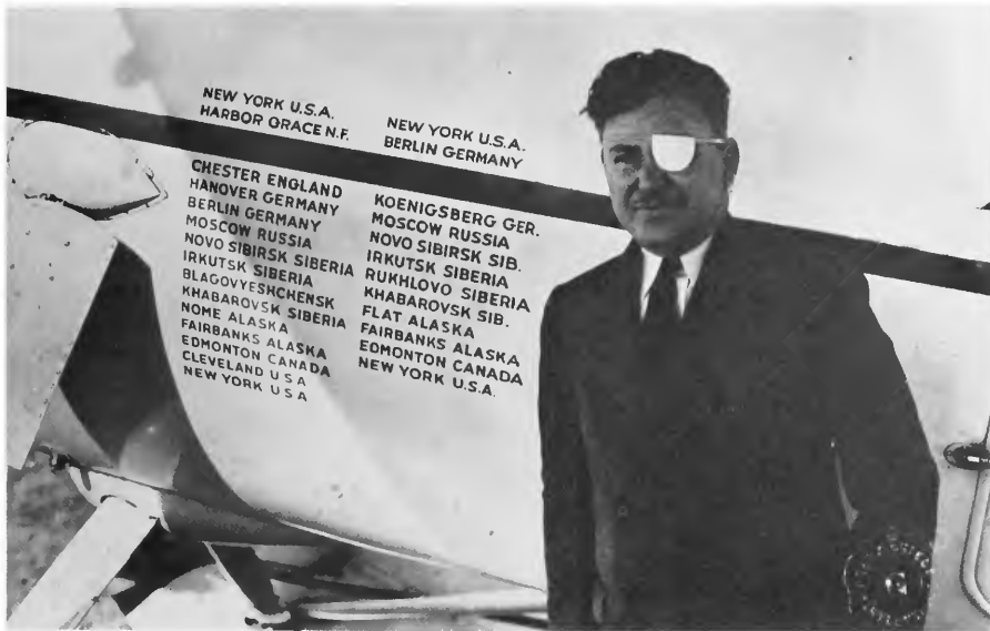
FIGURE 93.—Post stands beside the itinerary of his around-the-world record flights painted on the Winnie Mae (1931 left, 1933 right). Note the cracks in the fuselage paint that were aggravated by the low temperatures of the stratosphere (as low as -70^{\circ}\text{F} ). (Courtesy Phillips Petroleum Company.)
