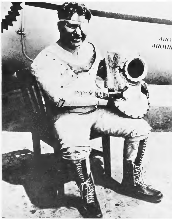
FIGURE 77.—Wiley Post dons the third and final version of his pressure suits. The pressure gauge held in his right hand was used to monitor the suit pressure. Just below the left inner knee is seen the outflow port to which the gauge could be attached. Note the ingenious joints at the knee and elbow portions of the suit, facilitating limb motion. Post had on his traditional “long-johns” under the suit. The suit was entered at the neck. Photograph taken at Dayton, Ohio, August 1934. The glass faceplate is screwed onto the helmet. The Pure Oil Company insignia is just forward of the door, but the edge of the E had been deleted from the picture at the request of a later sponsor. (Courtesy Goodrich Company.)
