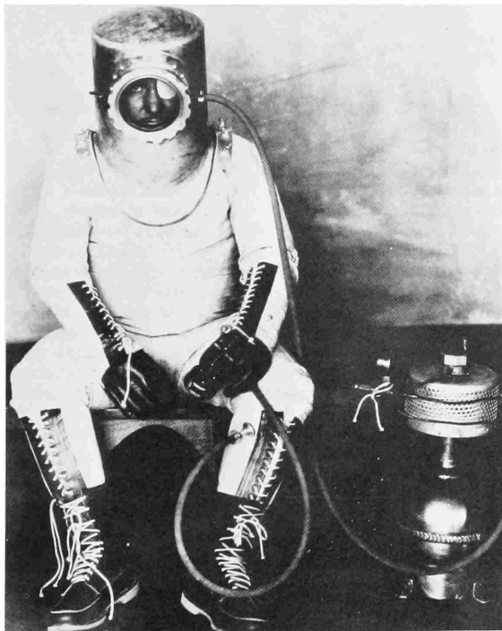
FIGURE 75.—The complete pressure-suit ensemble used by Wiley Post for inflight studies. Liquid oxygen is in the spherical tank. The liquid-to-gas conversion unit is attached to the top of the tank. The oxygen-inflow tube leads from the converter to the left side of the helmet. In Post's left hand is the outflow pressure-monitoring gauge. A second gauge on the oxygen converter gives inflow pressure information. Photograph made at Wright Field, August 27, 1934. (Courtesy U.S. Air Force.)
