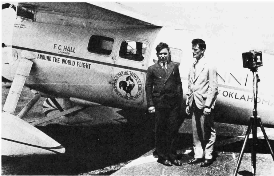
FIGURE 20.—Post and Gatty pose with the Winnie Mae just prior to the 1931 around-the-world flight. The aircraft sports the Pathé News emblem, and the on-board radio transmitter and receiver can be seen through the fuselage windows. On the tripod to the right is a contemporary radio microphone. (Courtesy Lockheed Aircraft Company.)
