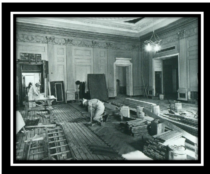
Figure 89: Carpenters laying down new floors in the State Dining Room in 1952.
