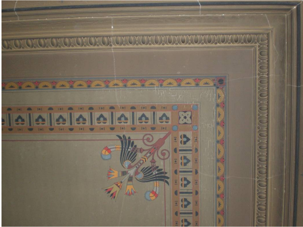
Figure 2.14: Detail of stenciling on corner of ceiling
