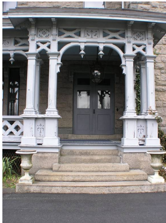
Figure 1.28: Paired posts of the verandah at the front entrance
