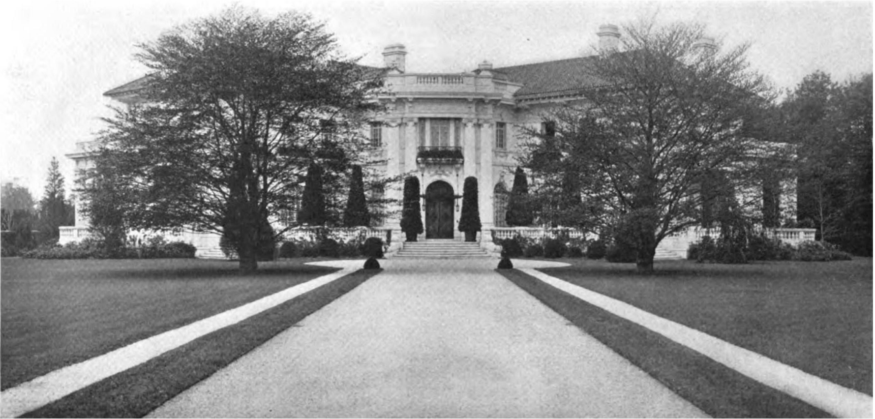
Whiteholme, Newport, Rhode Island. [From Herbert Croly, " A New Use of Old Forms: Two Houses by Mr. John Russell Pope ," Architectural Record Vol. 17 No. 4, April (1905): 282. Courtesy of the University of California, California]
