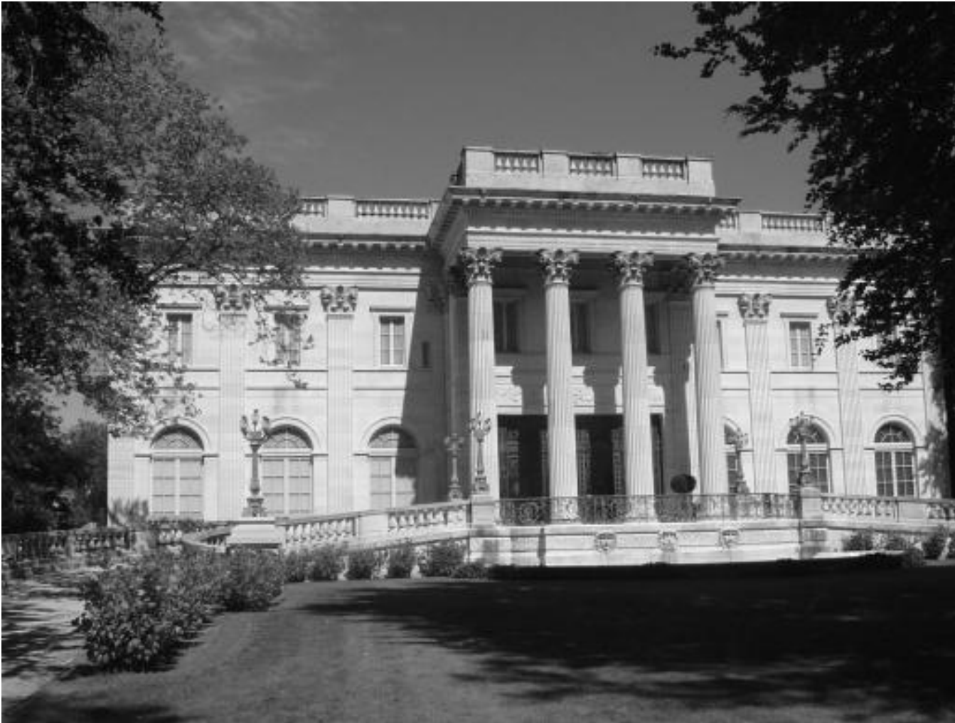
Marble House, Newport, Rhode Island. [Photograph by the author, 2009]
