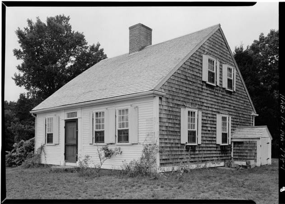
Figure 3. Gormley House, Herring Pond Road, Wellfleet, Massachusetts, built c. 1830. A typical Cape Cod house with peaked roof, central chimney, and shingled sides. LOC HABS, MASS,1-WEL,7- .
