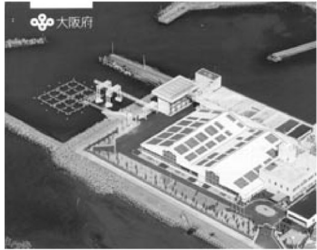
Figure 5. Example of Prefectural Farming Fisheries Center (1991), Osaka Fisheries Experimental Research Station, Tanigawa, Osaka Prefecture. Note outdoor tanks for Nannochloropsis and rotifer culture. Facility includes multispecies spawning tanks and larval rearing tanks (100-300 m 3 ). Facility also includes outdoor rearing pens and indoor offices and research laboratories. Note seashore tripods and seawall that typifies most of Osaka Bay's intertidal habitats.
