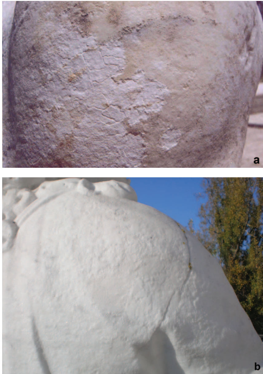
FIGURE 4. Surface conditions left by two different cleaning methods: (a) application of a biocide and gentle brushing (roughly 30 \times 40 cm area) and (b) aggressive grit blasting (area about 40 \times 50 cm).
