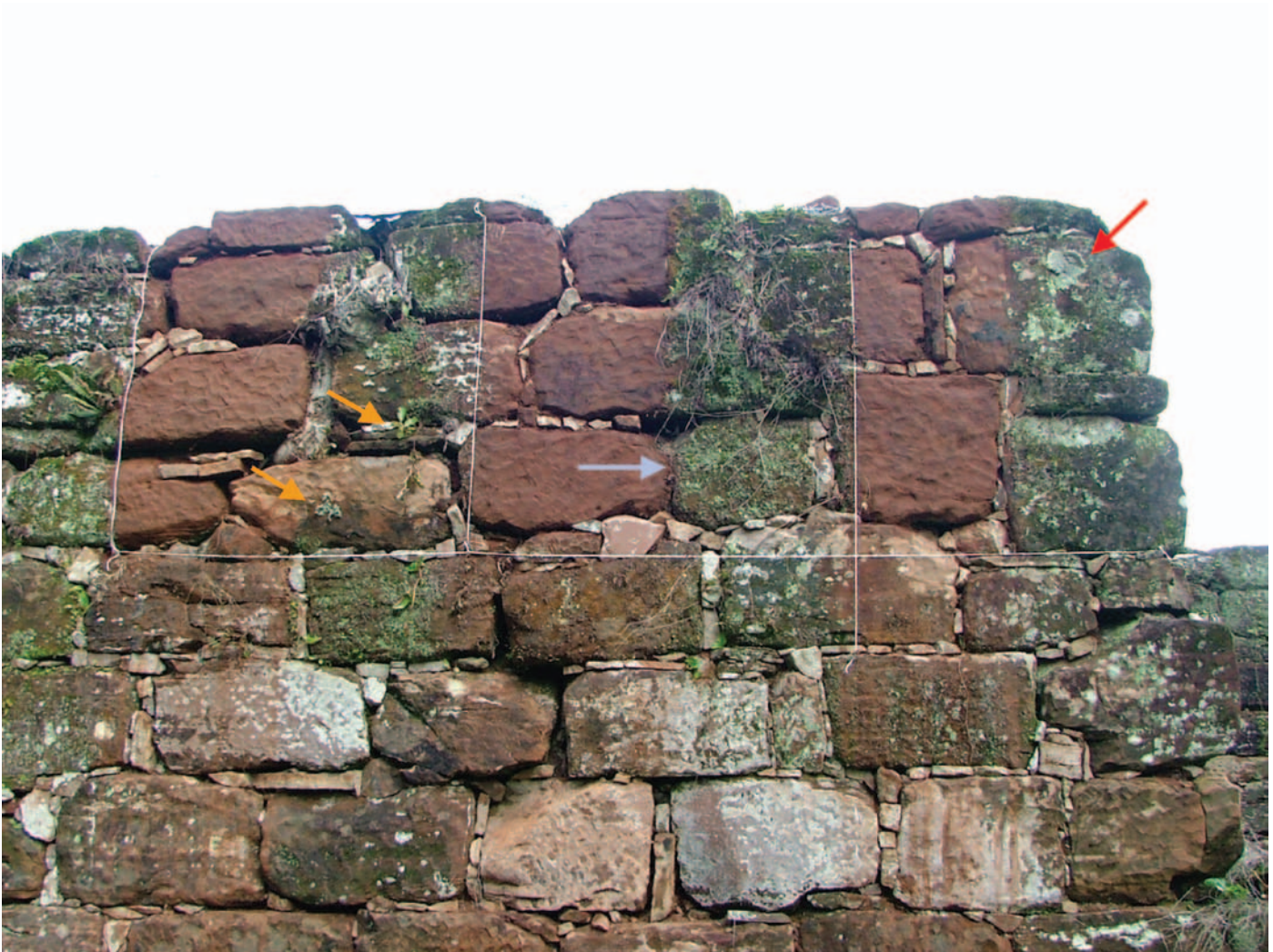
FIGURE 3. View of the north side of the wall where the passive control systems were installed on the top. The left area is below lead strips, the middle area is below zinc mesh, and the right area is below brass mesh (photo taken in May 2007). The left half of each area had been cleaned at the beginning of the experiment; the right half was left uncleaned and served as a control. The upper orange arrow points to a small plant, and the lower one points to a hepatica. The blue arrow points to a moss- and hepatica-covered block. The red arrow points to a detaching lichen.
