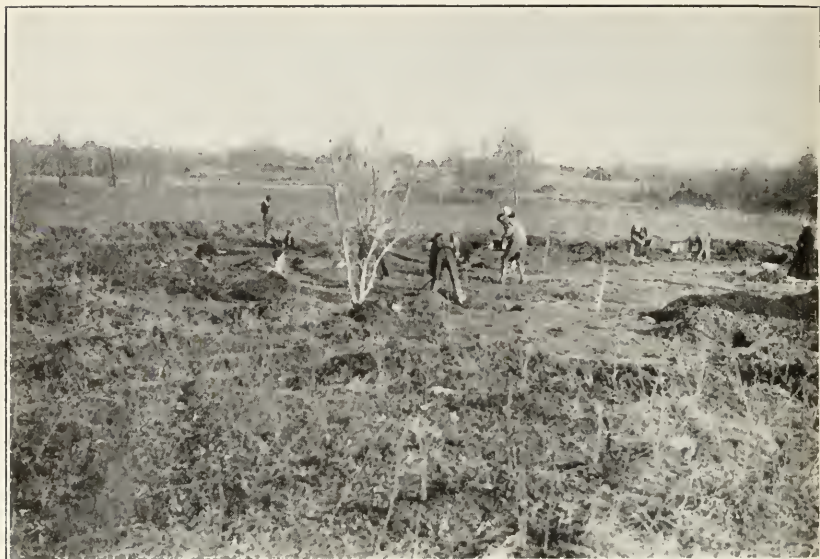
a , EXCAVATION OF HOUSE RING NO. 1
