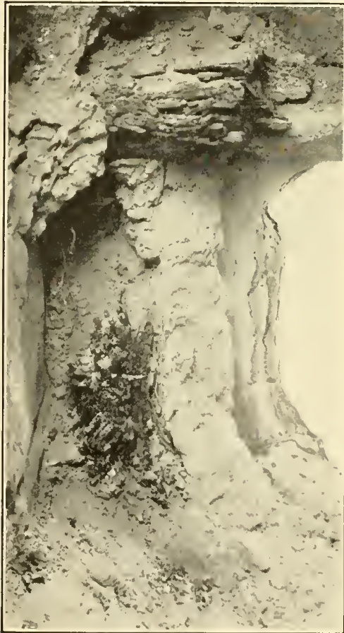
b, Doorway from passage side. Note timbers for passage covering, also plaster reducing size of doorway
