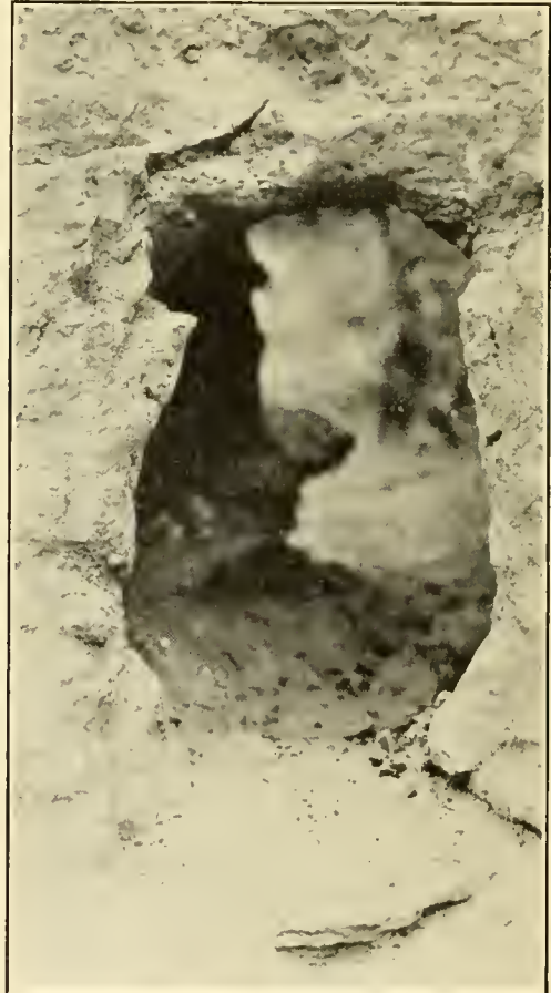
c, Doorway from room side. This picture shows the manner in which the original opening was later reduced in size by use of plaster
