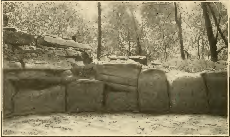
a , The small slab in the middle wall covers the ventilator passage in the Cave 3 kiva, Cottonwood Canyon
