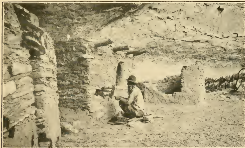
b , Repairing broken walls in Cave 3, Cottonwood Canyon
