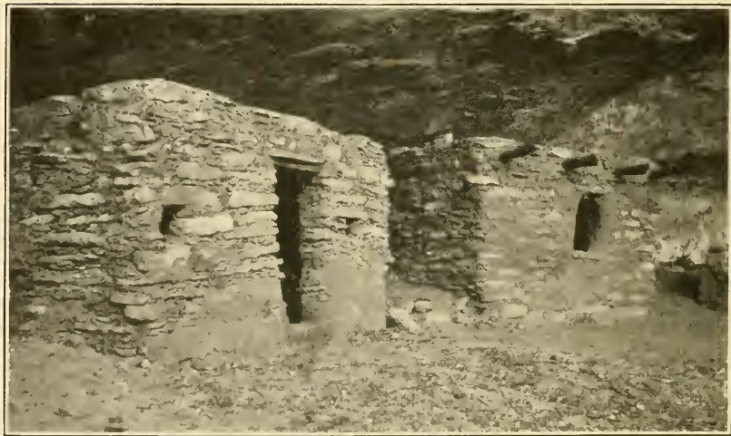
b , Rooms 2 and 3, Cave 3, Cottonwood Canyon, showing doors and windows
